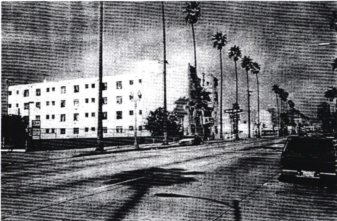
Photo 3: Apartment building on Flower Street north of the Harbor Freeway overpass.
