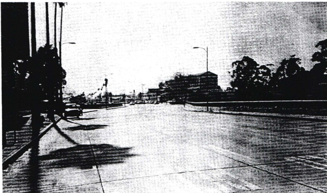
Photo 4: View looking south on Flower Street at Harbor Freeway overpass.
