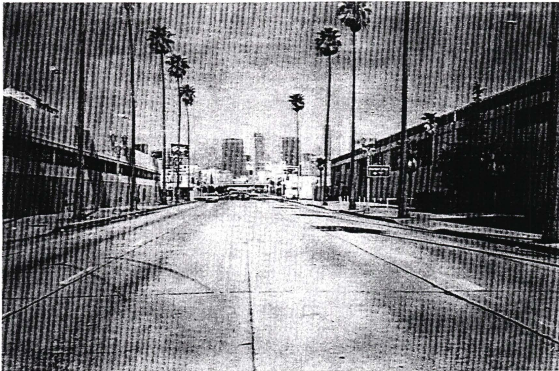
Photo 1: View looking north on Flower Street.
