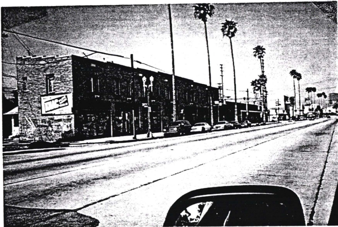
Photo 6: Commercial building (upper floor residential uses) on west side of Flower Street.
