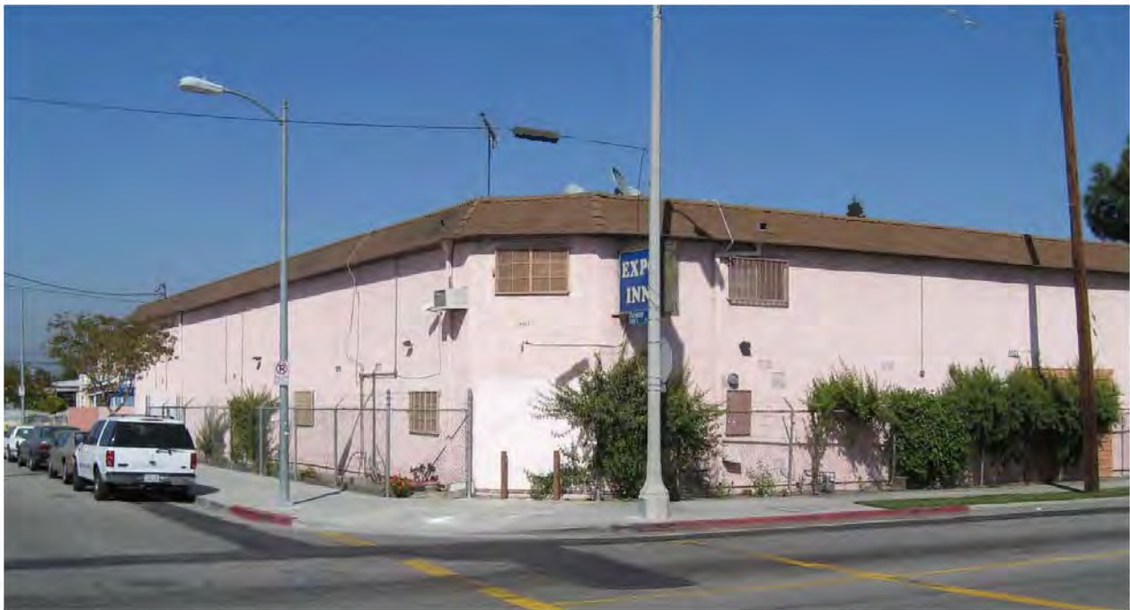
Image 12. View facing northeast, looking across Exposition Boulevard, toward the Expo Inn Motel on the northeast corner of the intersection of Farmdale Avenue and Exposition Boulevard.
