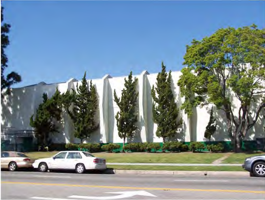
Image 19. Auditorium's south façade facing Rodeo Road. This view shows extant and original "fins" of vertically oriented stucco-clad steel trusses bracing the sides of the Auditorium. Photo taken looking north from Rodeo Road.
