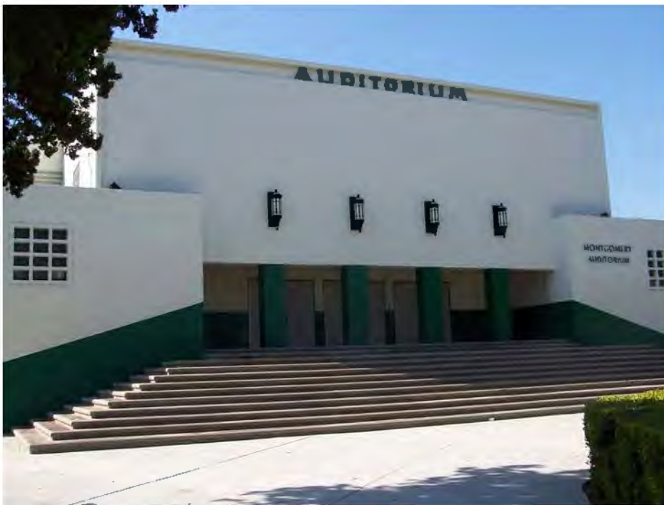
Image 18. Auditorium's east façade. This free-standing building is south of and separated by the Administration Building by a sequence of one-story classrooms; the roofs of these wide-span rooms employ unusual cantilevered trusses. The Auditorium visually anchors the south end of the primary façade. Photo taken looking northwest from Farmdale Avenue.
