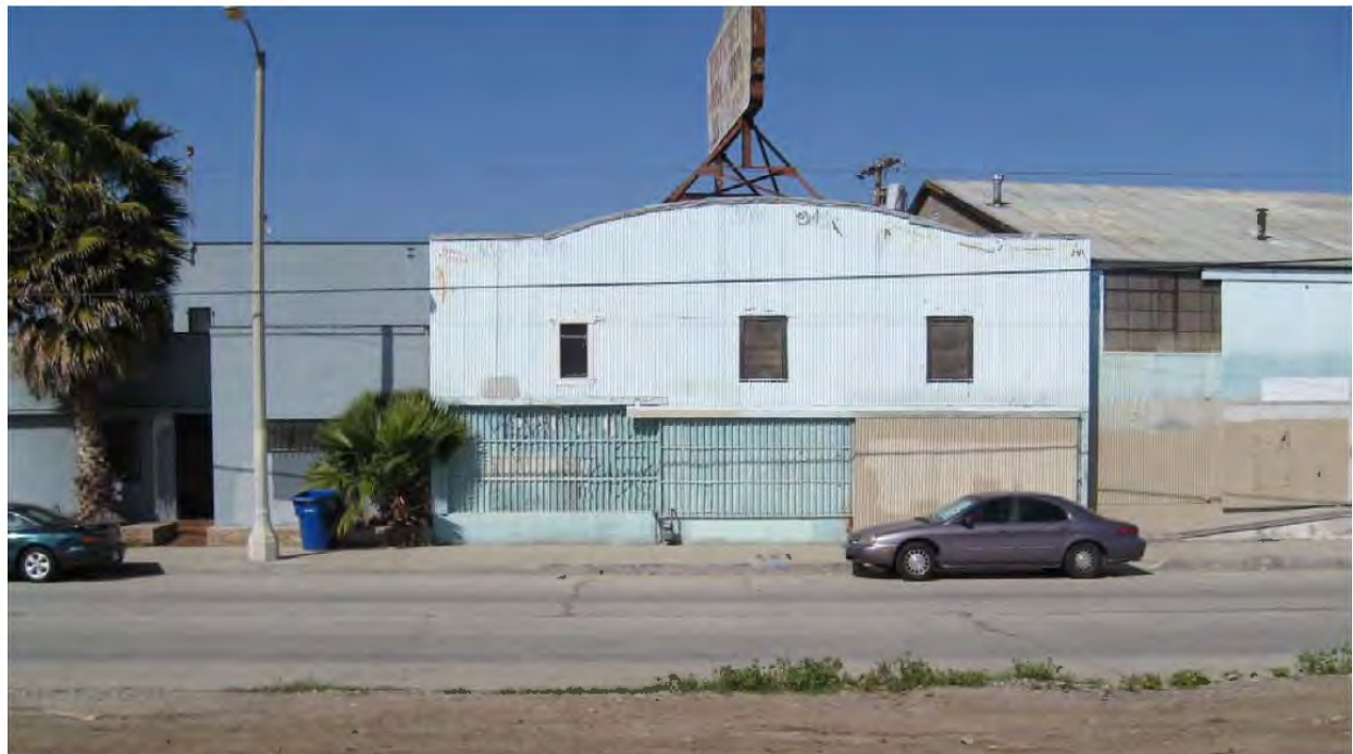
Image 6. View facing north, looking across Exposition Boulevard from the northern edge of Dorsey High School, to the west of the intersection of Farmdale Avenue and Exposition Boulevard.
