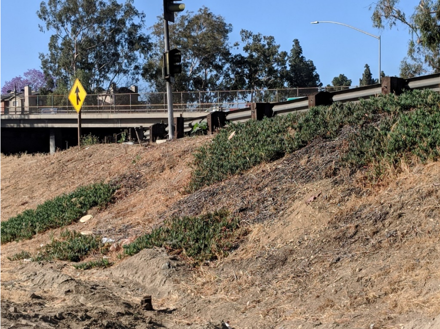
Figure 4 - Existing landscaping along slope
