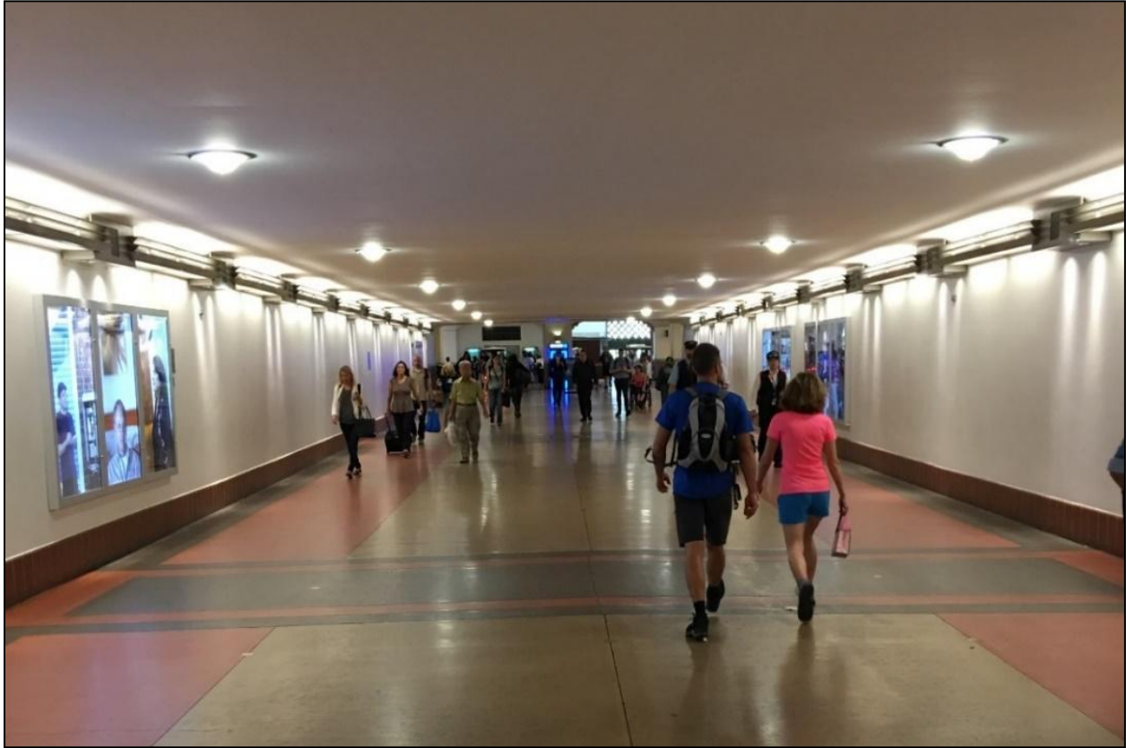
Figure 4-18. Key View #6c – Los Angeles Union Station Pedestrian Passageway (view looking west from passageway toward passageway entrance)
