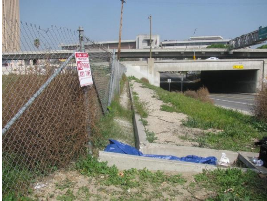
Photograph 7. Two-foot-wide drainage ditch along the fence line on the corner of Commercial and Center Streets, looking north
