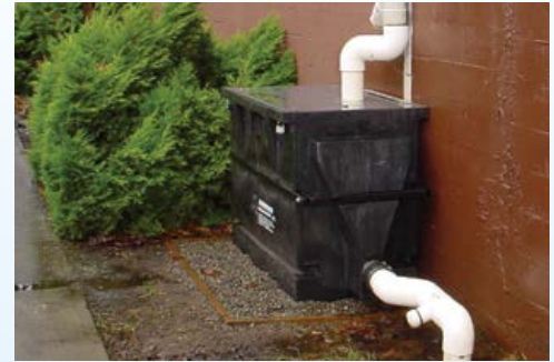
DownSpout StormFilter
