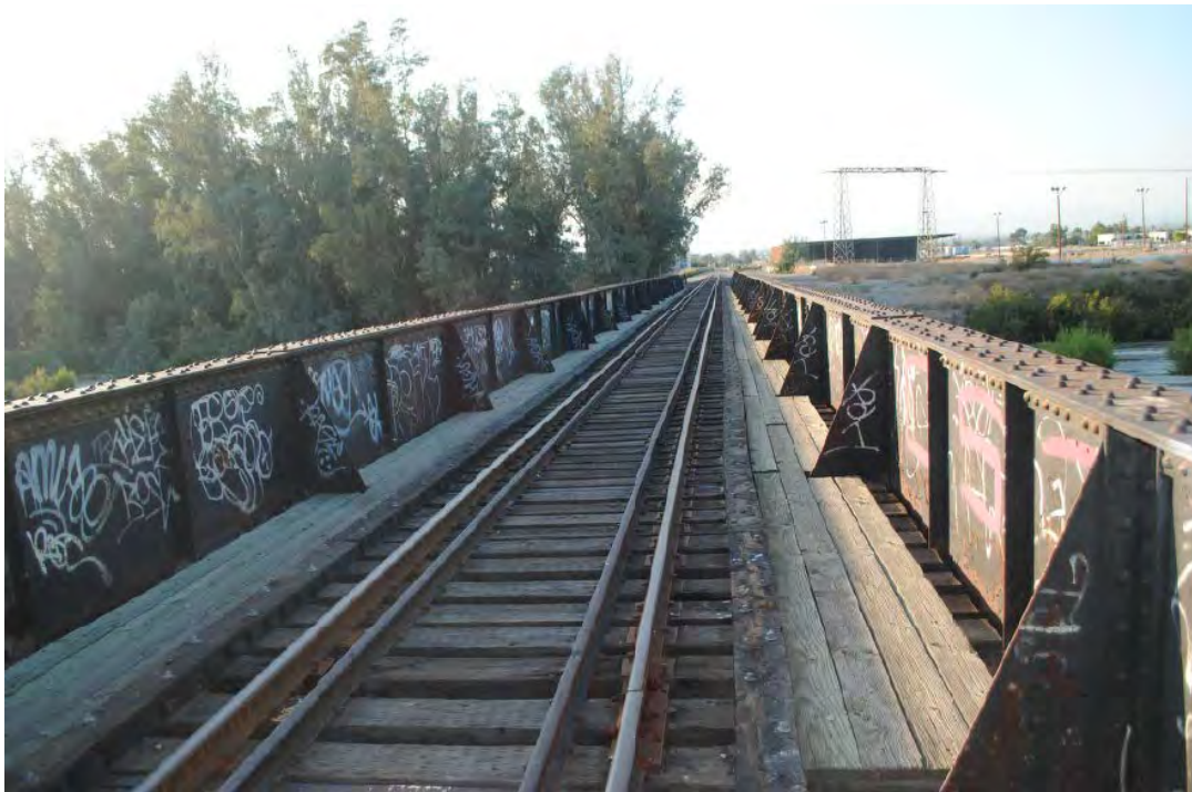
Figure 2: Existing AT&SF Bridge 3.4
