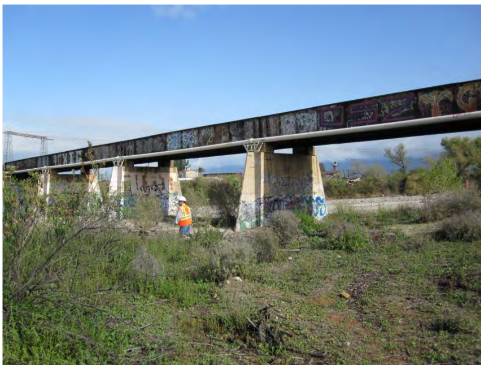
Figure 1: Santa Ana River, AT&SF Bridge 3.4 Downstream Face
