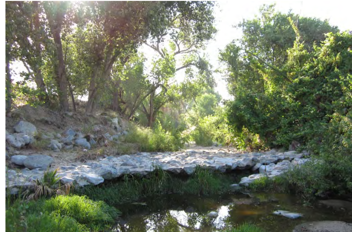
Photograph 4: View looking east within Zanja Channel, approximately 300 meters east of the confluence with the Santa Ana River.
