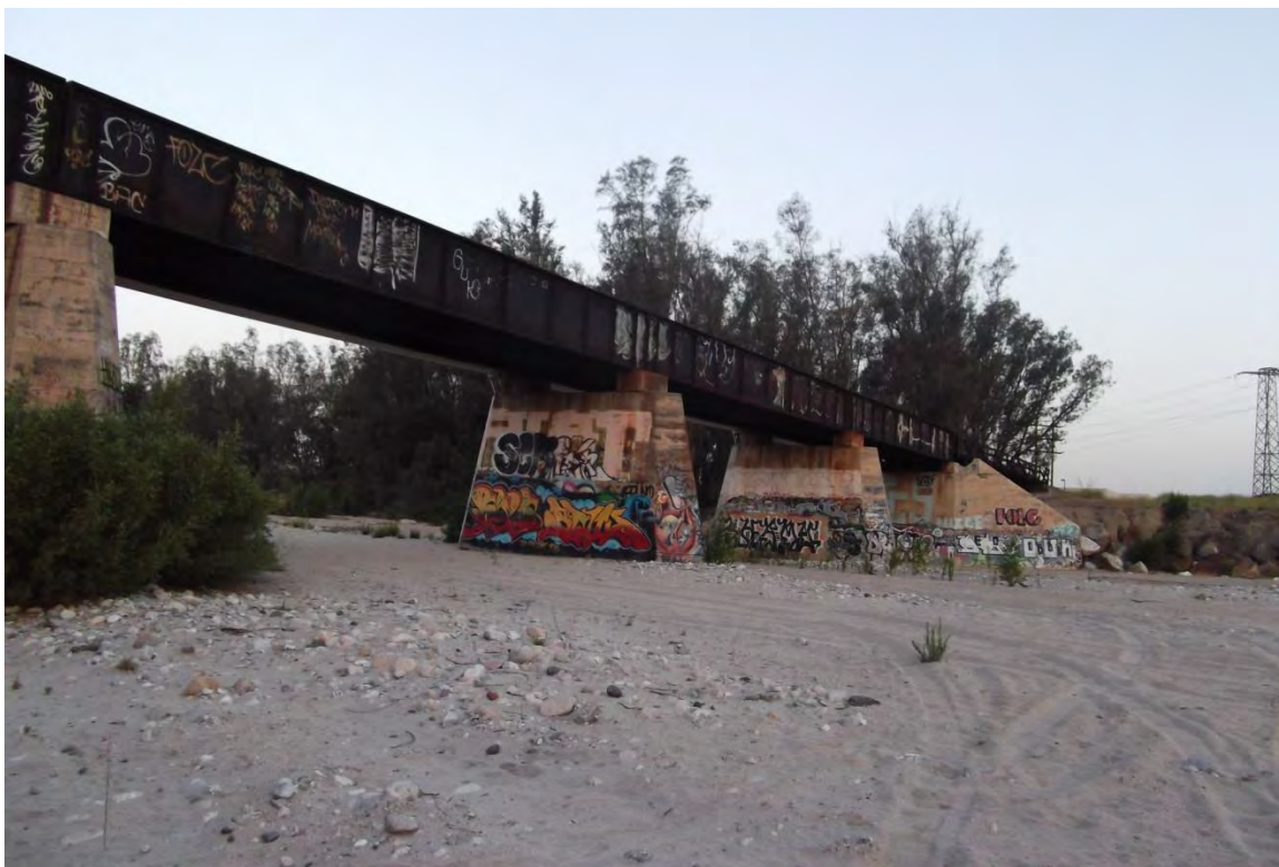
Photo 2. Standing on east side of bridge looking north/northwest.
