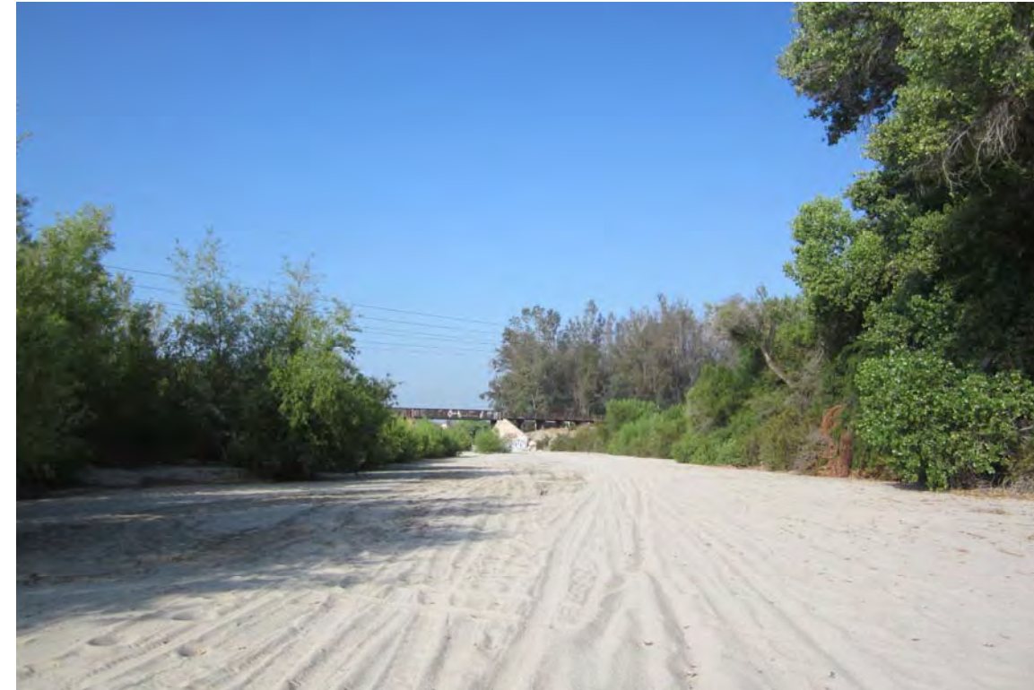
Photograph 2: View looking southwest at the Santa Ana River, north (upstream) of the railroad bridge crossing.
