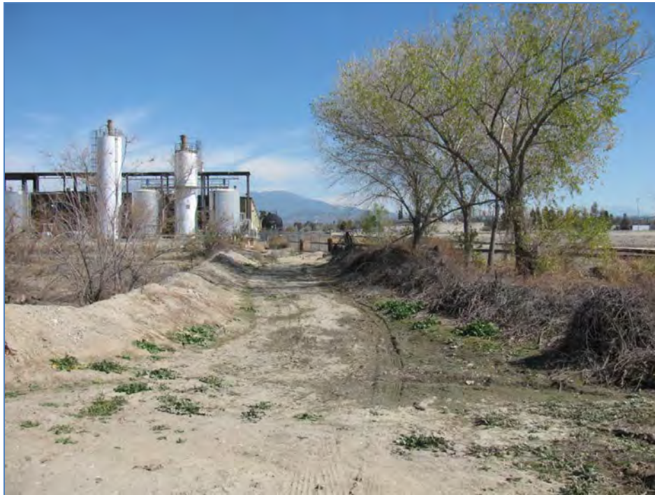
Photograph 16. Manufactured earthen berm separating the storm water runoff (soil pits #1 and #2) from Zanja Channel.
