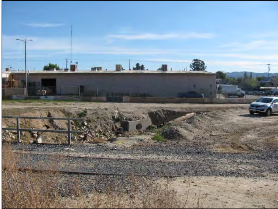
Photograph 13. Mill Creek Zanja. Westerly view.
