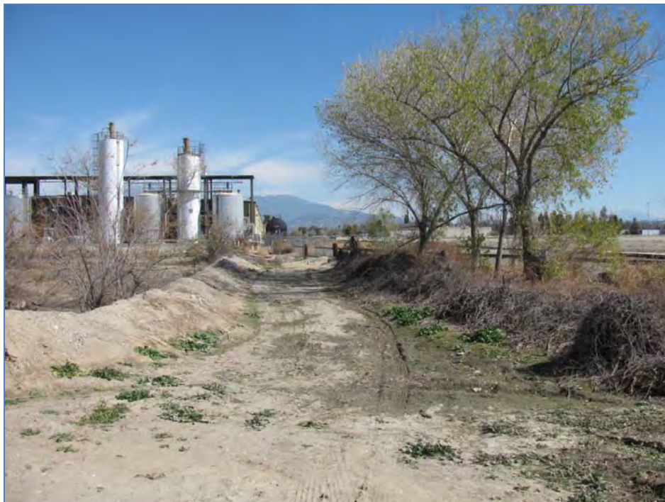
Photograph 16. Manufactured earthen berm separating the storm water runoff (soil pits #1 and #2) from Zanja Channel.
