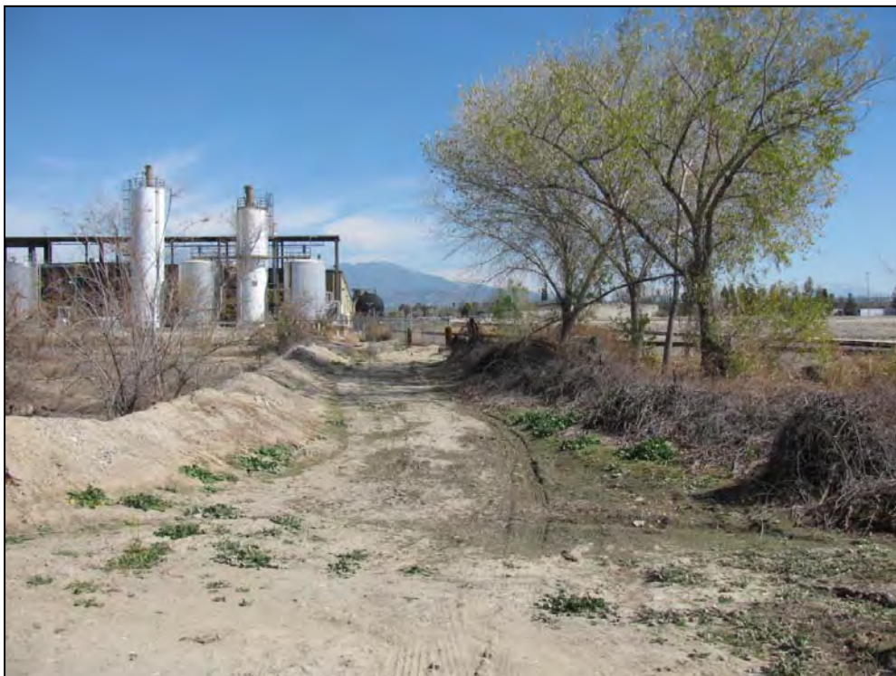
Photograph 18. Manufactured earthen berm separating the storm water runoff (soil pits #1 and #2) from Zanja Channel .
