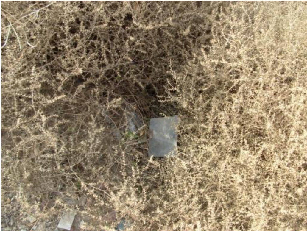
MP 2.4, 22-inch x 13-inch CMP
