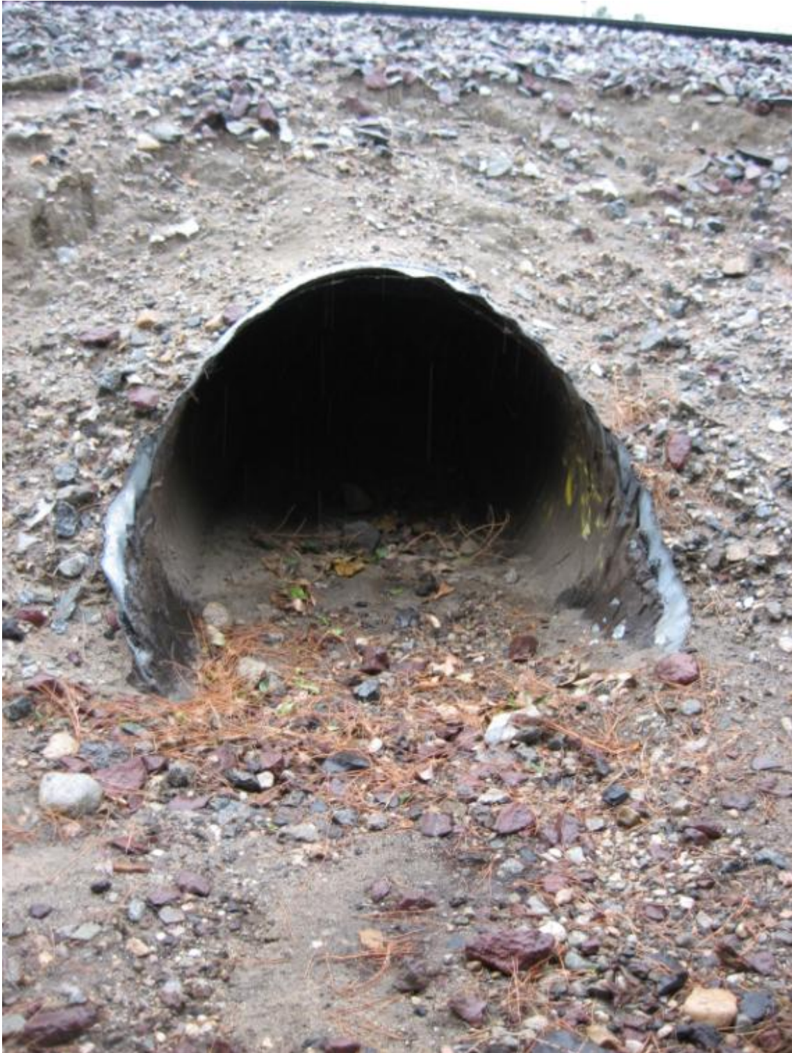
MP 2.25, 36-inch CMP (no. 1)
