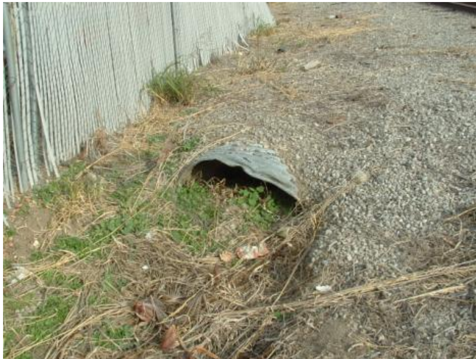
MP 4.2, culvert (no. 5)
