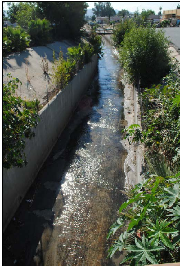
Figure 1: Existing AT&SF Bridge 1.1- Looking Downstream
