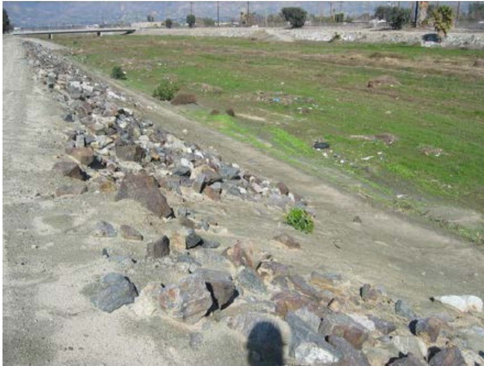
Figure 1: Twin Creek Downstream of AT&SF Bridge 2.2
