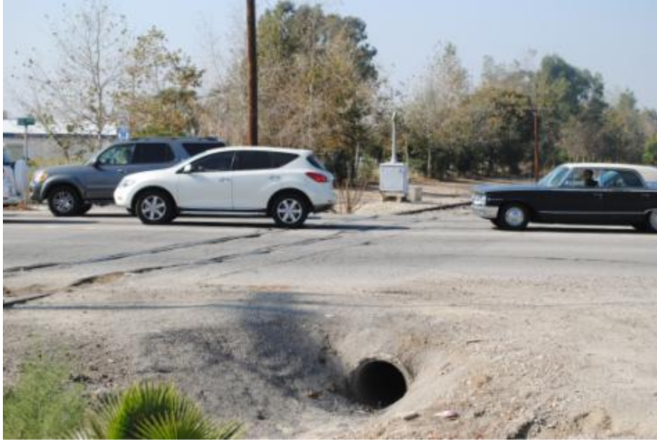
MP 7.8, 24-inch culvert (no. 3)
