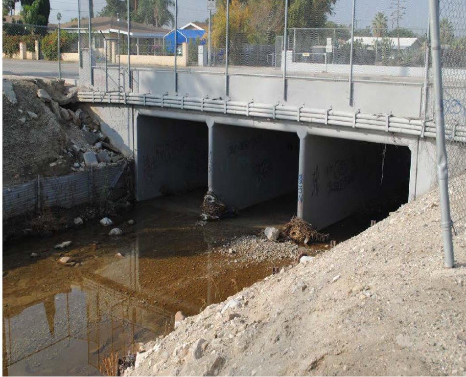
Photo 5: Richardson Bridge – Looking downstream
