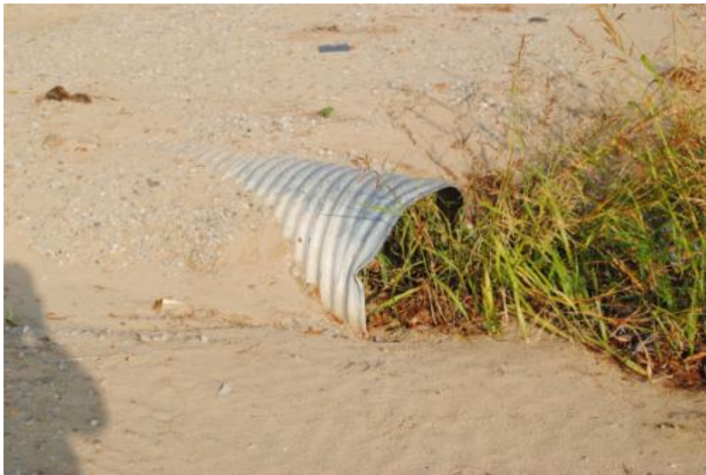
MP 4.2, 36-inch culvert (no. 1)
