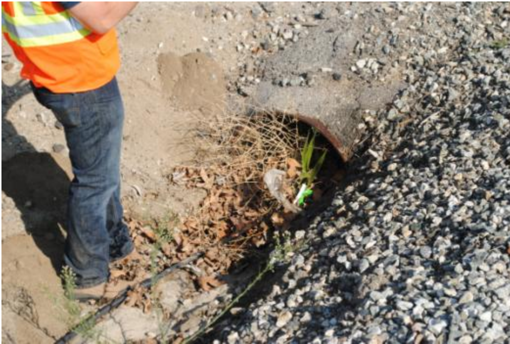
MP 8.2, 12-inch CMP (no. 2)
