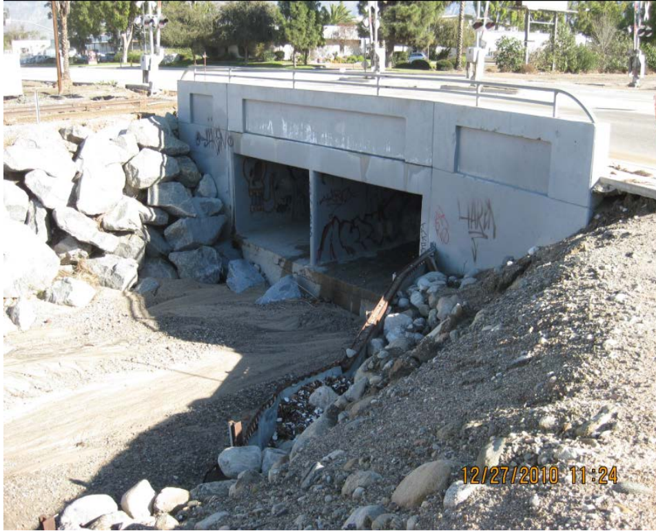
Photo 3: Tippecanoe Ave Culvert – Downstream Face
