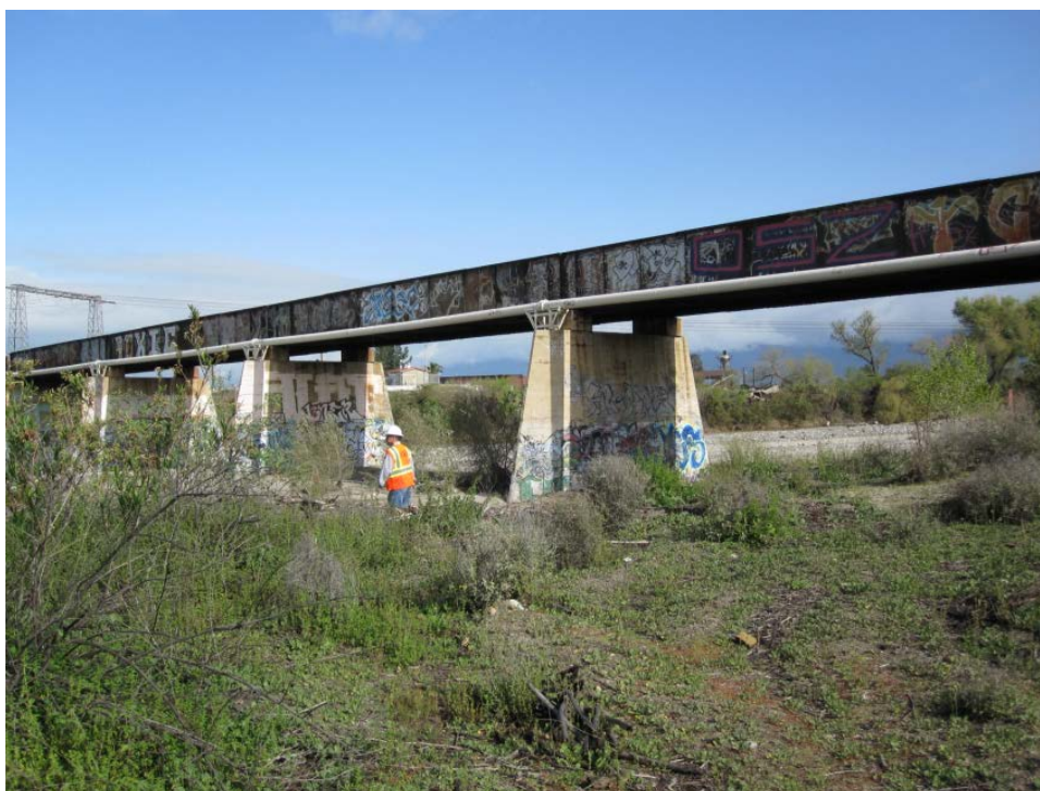
Figure 1: Santa Ana River, AT&SF Bridge 3.4 Downstream Face
