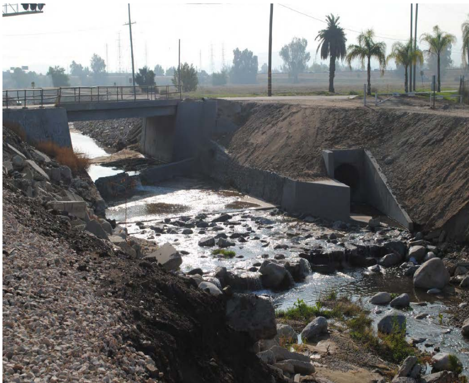
Photo 6: Mountain View Bridge – Looking upstream
