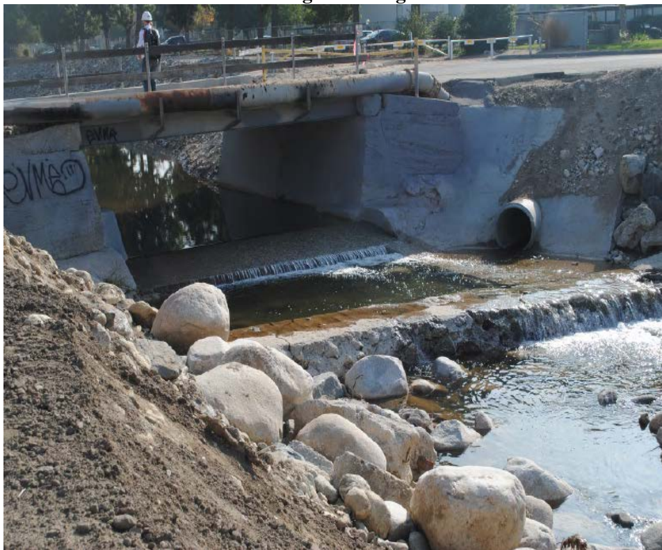
Photo 10: Bryn Mawr Bridge- Looking Upstream
