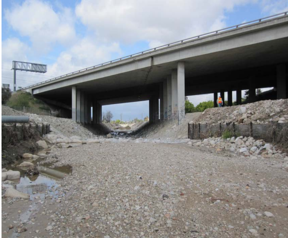
Photo 9: I-10 Bridge- Looking Downstream
