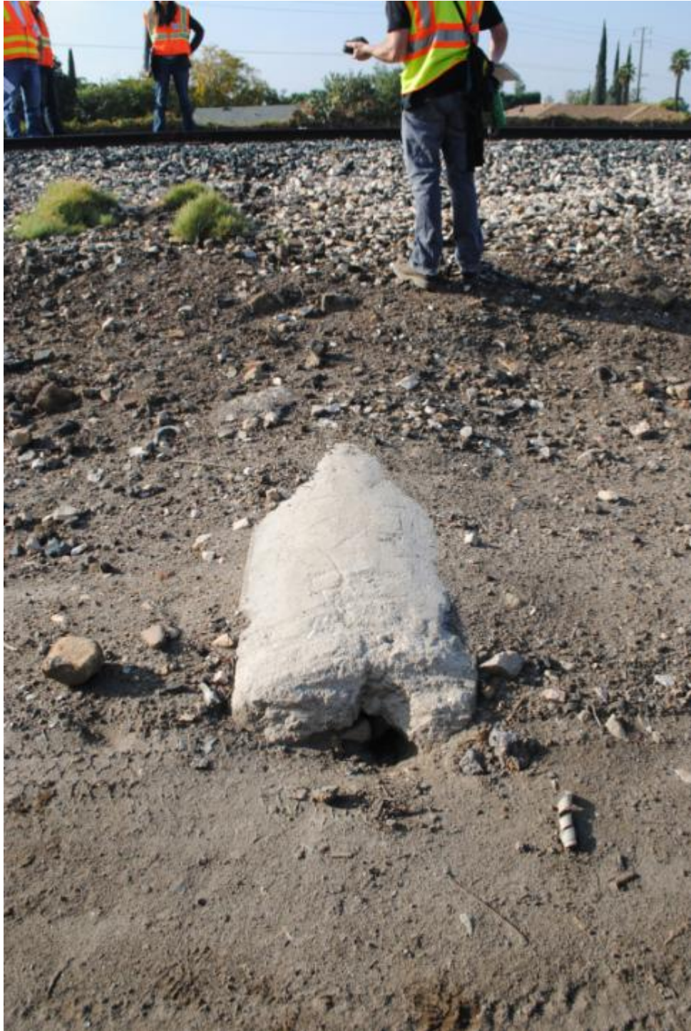
MP 5.1, buried culvert (no. 2)
