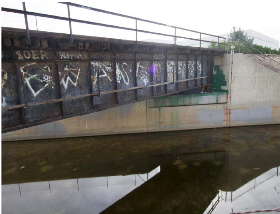
Figure 2: Existing AT&SF Bridge 2.2 – Downstream Face
