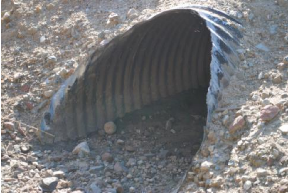
MP 2.25, 36-inch CMP (no. 2)
