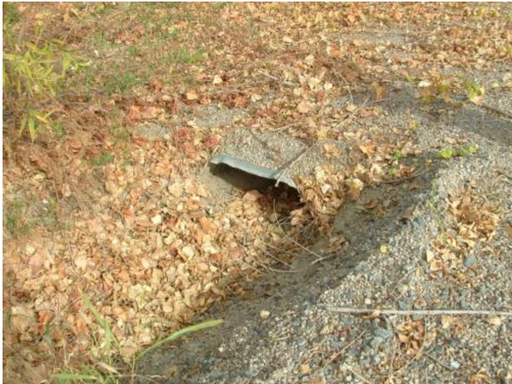
MP 3.9, culvert (no. 3)
