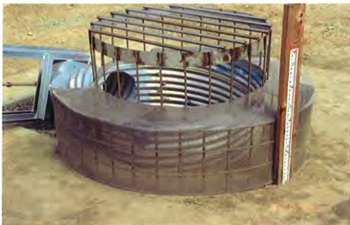
Figure 1 Example of Extended Detention Outlet Structure
