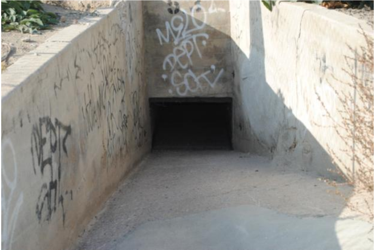
MP 5.2, 24-inch RCP (no. 2)
