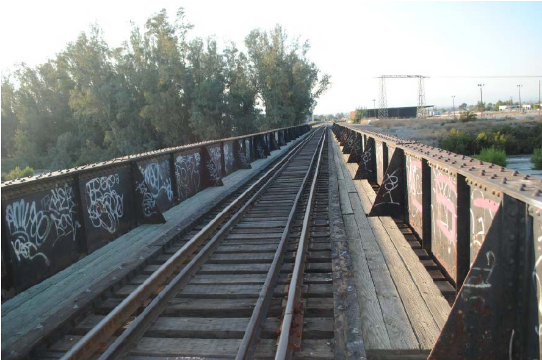
Figure 2: Existing AT&SF Bridge 3.4
