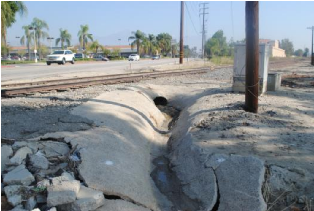
MP 7.4, culvert (no. 6)
