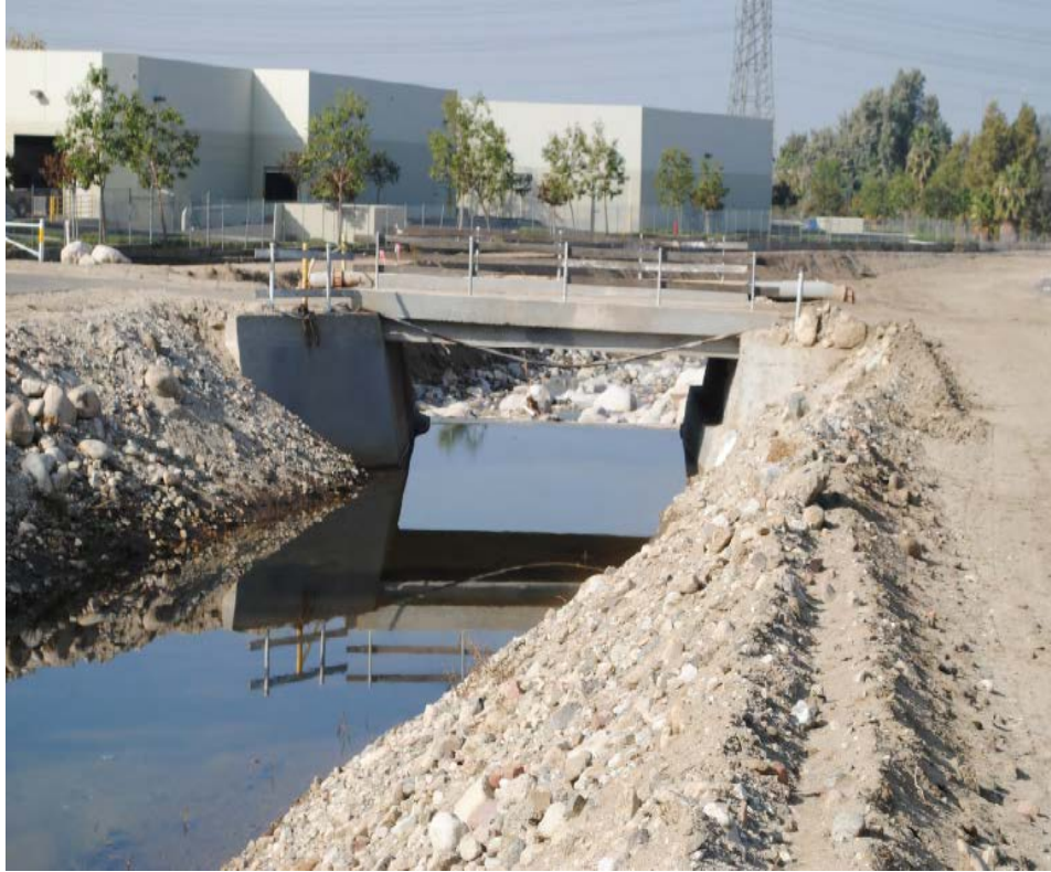
Photo 11: Bryn Mawr Bridge- Looking Downstream
