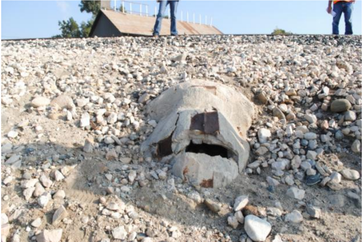
MP 5.1, buried culvert (no. 3)
