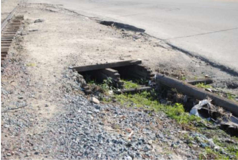
MP 7.4, 24-inch x 18-inch box culverts (no. 3)
