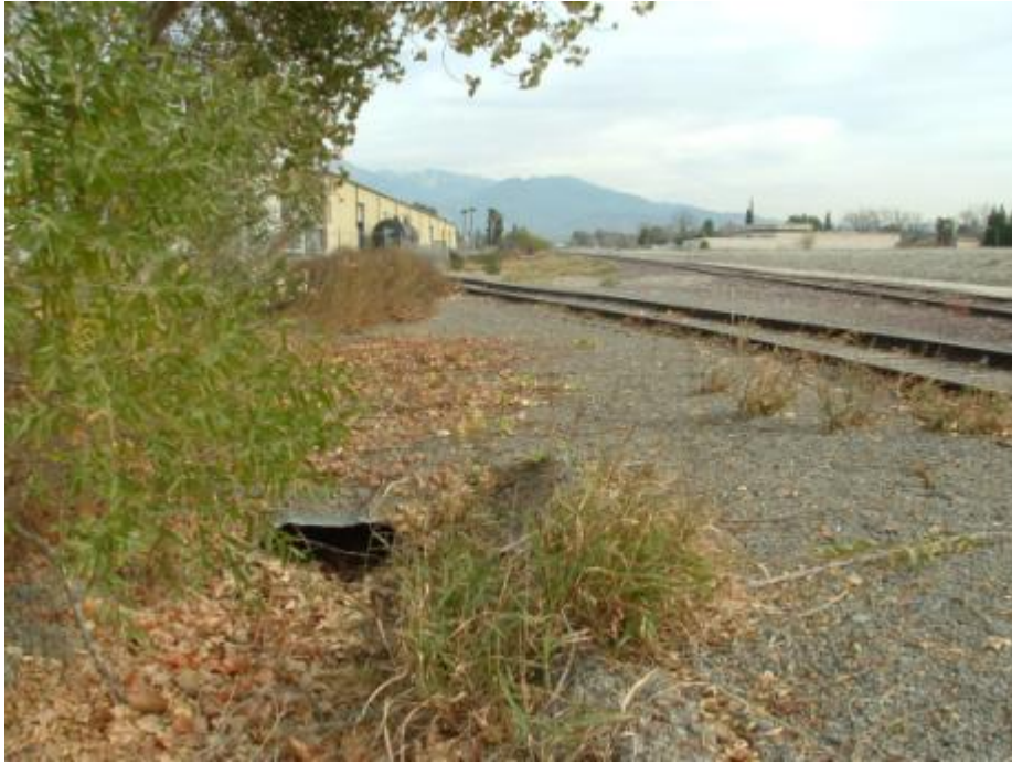
MP 3.9, culvert (no. 4)
