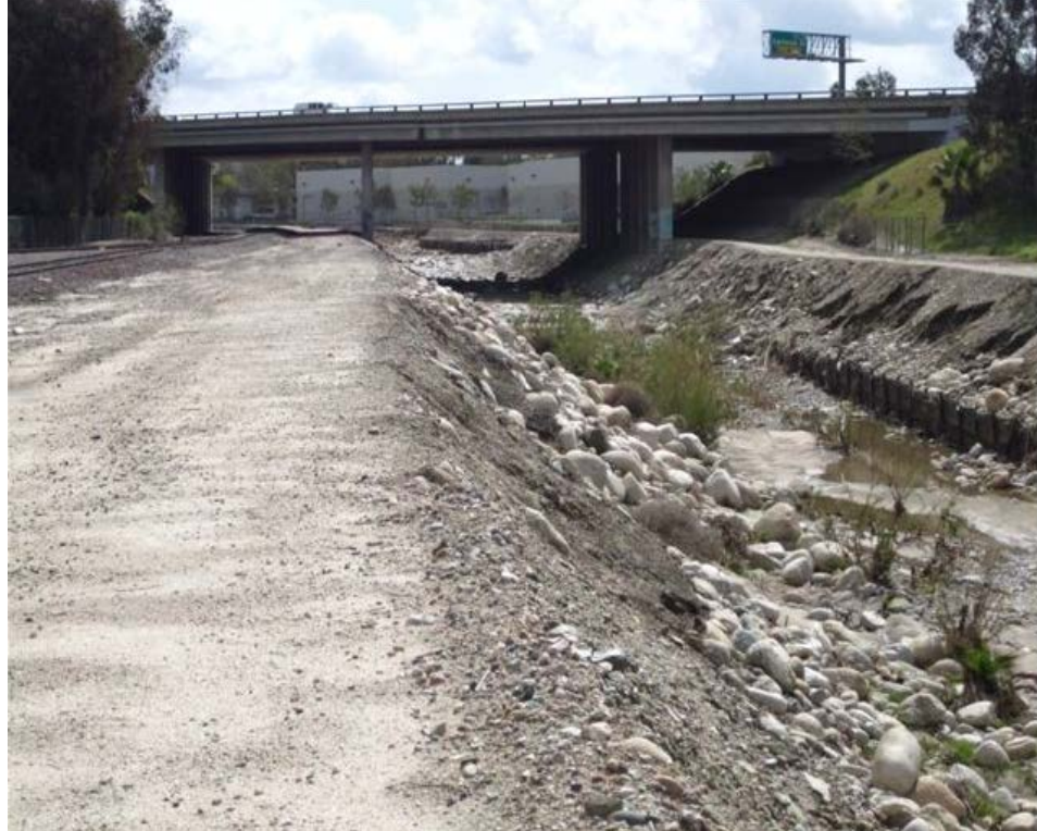
Photo 8: I-10 Bridge- Looking Upstream
