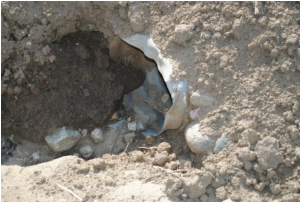
MP 6.05, 14-inch CMP
