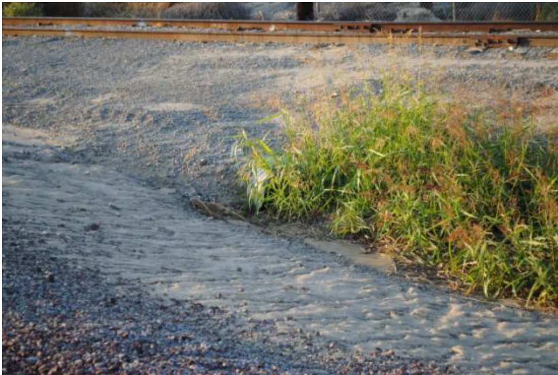
MP 3.9, culvert (no. 1)
