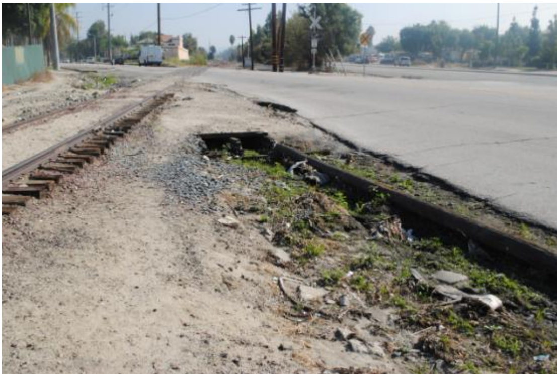
MP 7.4, 24-inch x 18-inch box culverts (no. 2)
