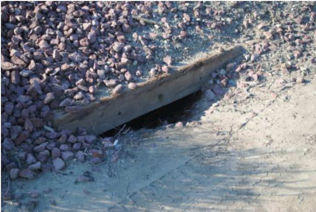
MP 2.6, 4-foot x 3-foot wood box buried (no. 2)
