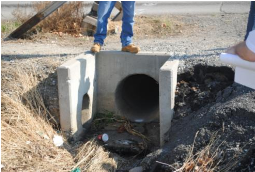
MP 7.8, 24-inch culvert (no. 2)
