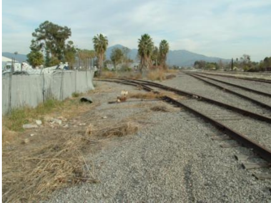
MP 4.2, culvert (no. 4)
