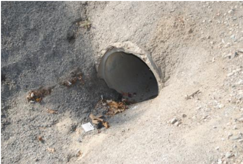
MP 7.8, 6-inch culvert (no. 4)
