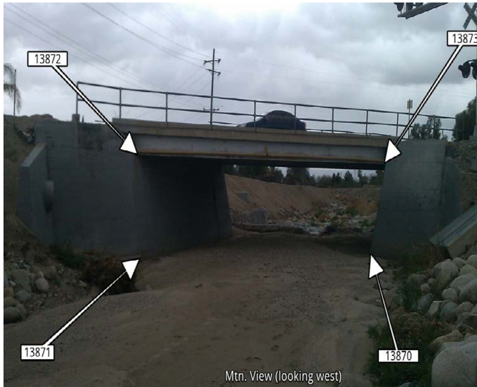
Photo 7: Mountain View Bridge – Looking downstream (from survey photo)
