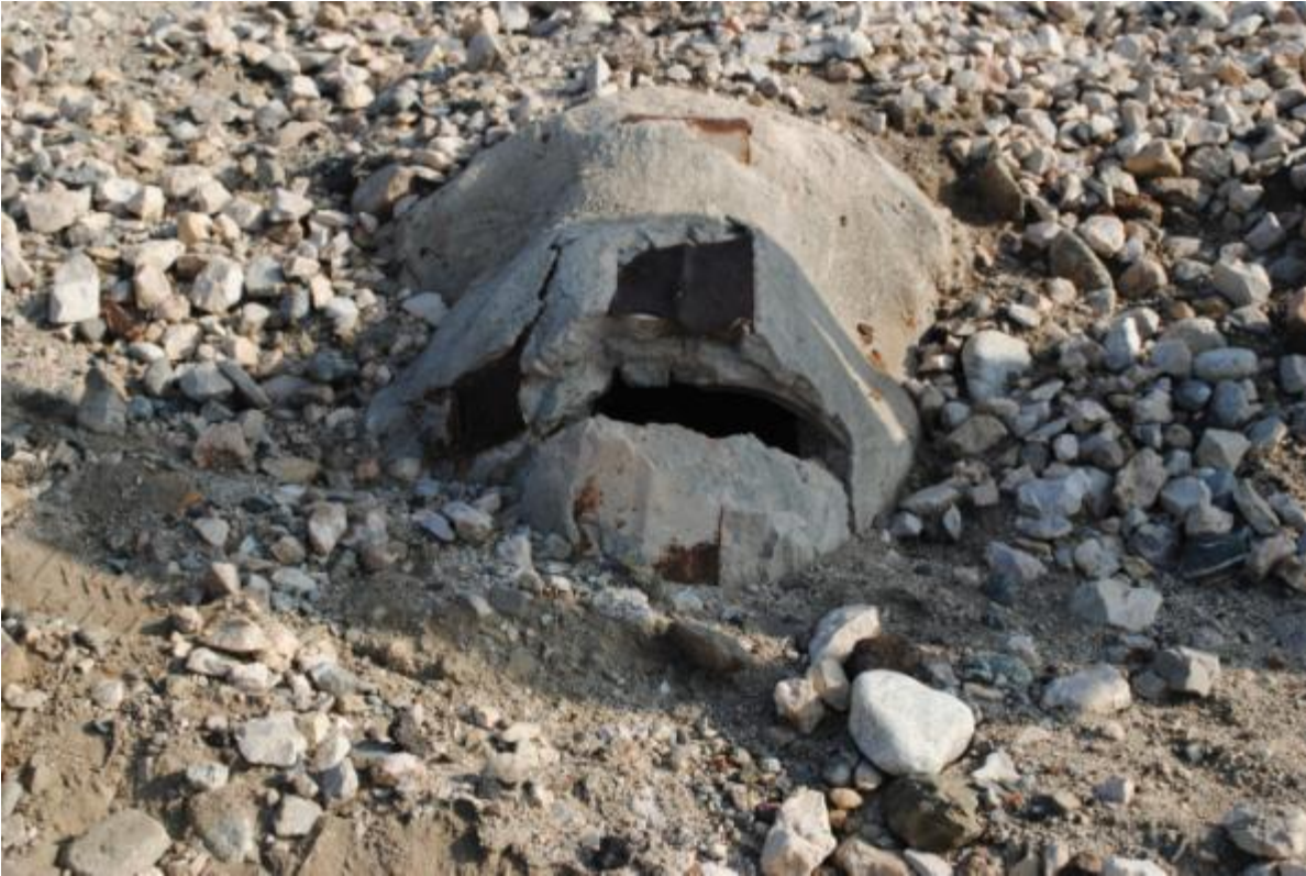
MP 5.1, buried culvert (no. 1)
