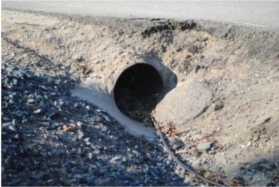
MP 8.2, 12-inch CMP (no. 1)
