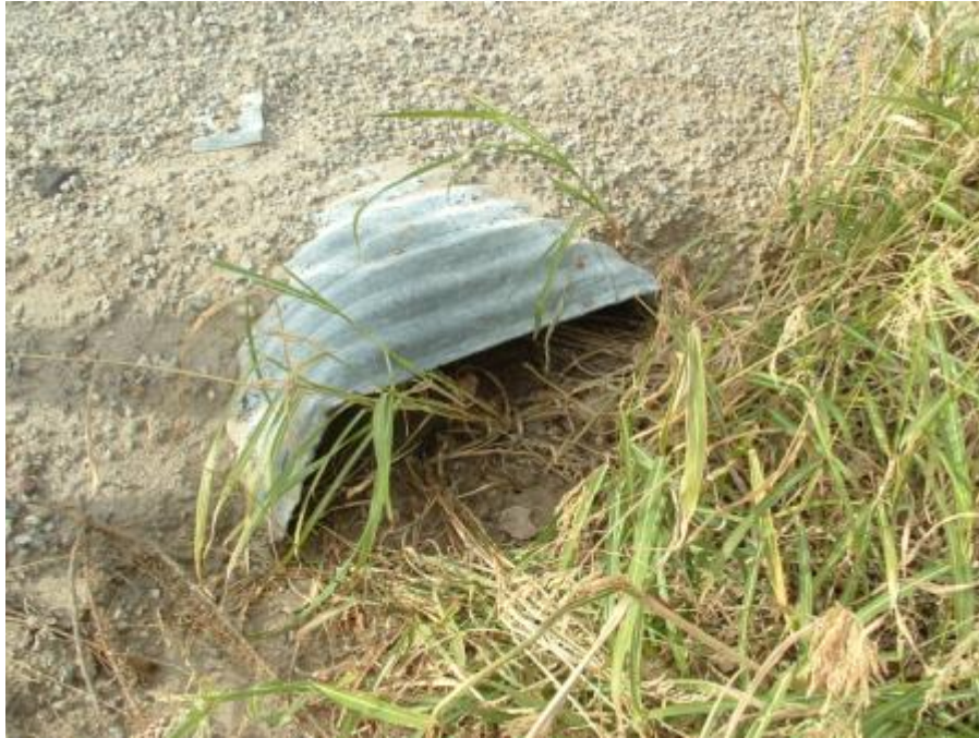
MP 3.9, culvert (no. 2)
