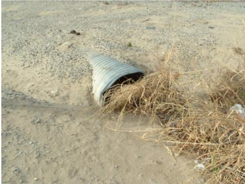
MP 4.2, 36-inch culvert (no. 2)
