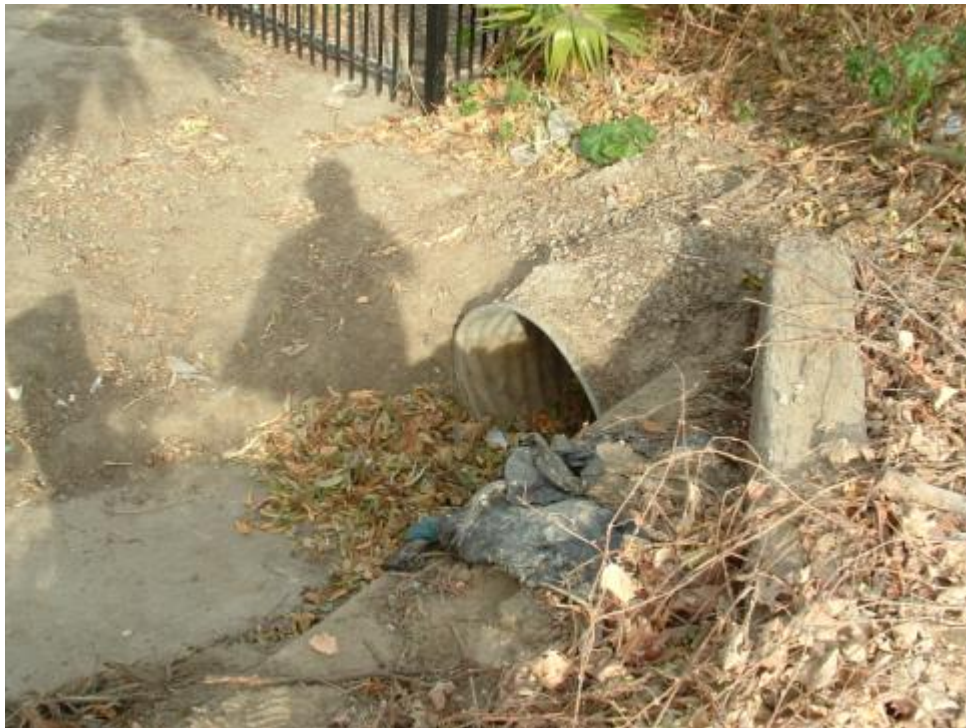
MP 4.2, culvert (no. 3)
