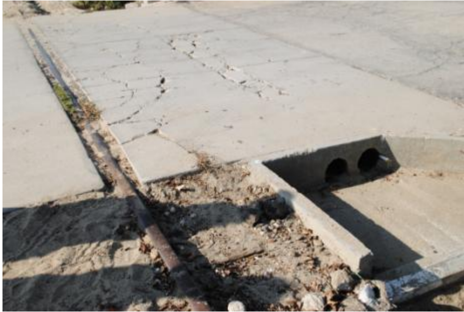
MP 7.8, 24-inch, 18-inch culverts (no. 1)
