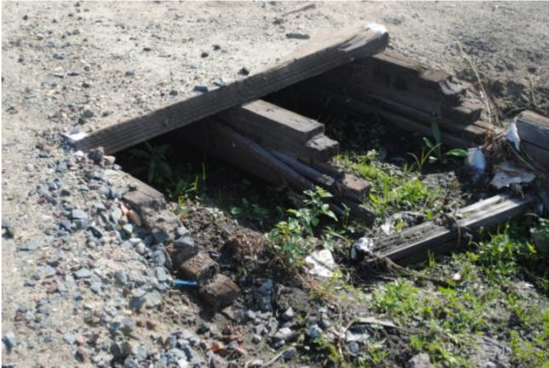
MP 7.4, 24-inch x 18-inch box culverts (no. 1)
