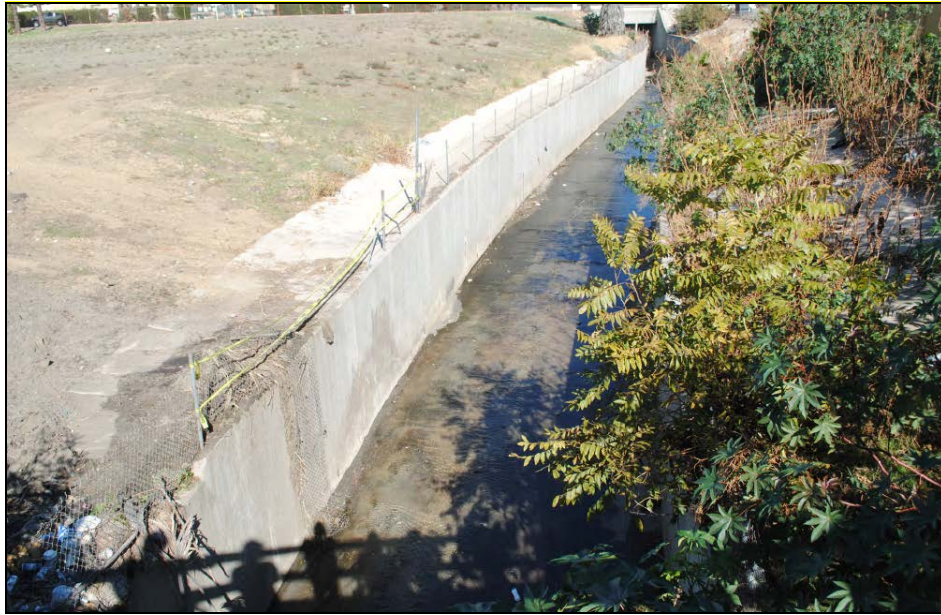
Figure 2: Existing AT&SF Bridge 1.1- Looking Upstream
