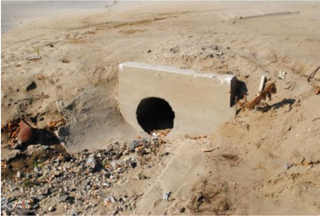
MP 7.4, culvert (no. 5)
