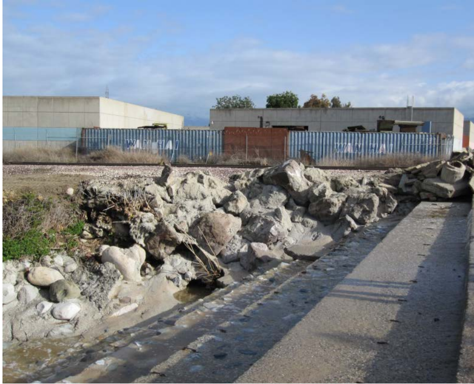
Photo 1: Gage Canal Drop Structure
