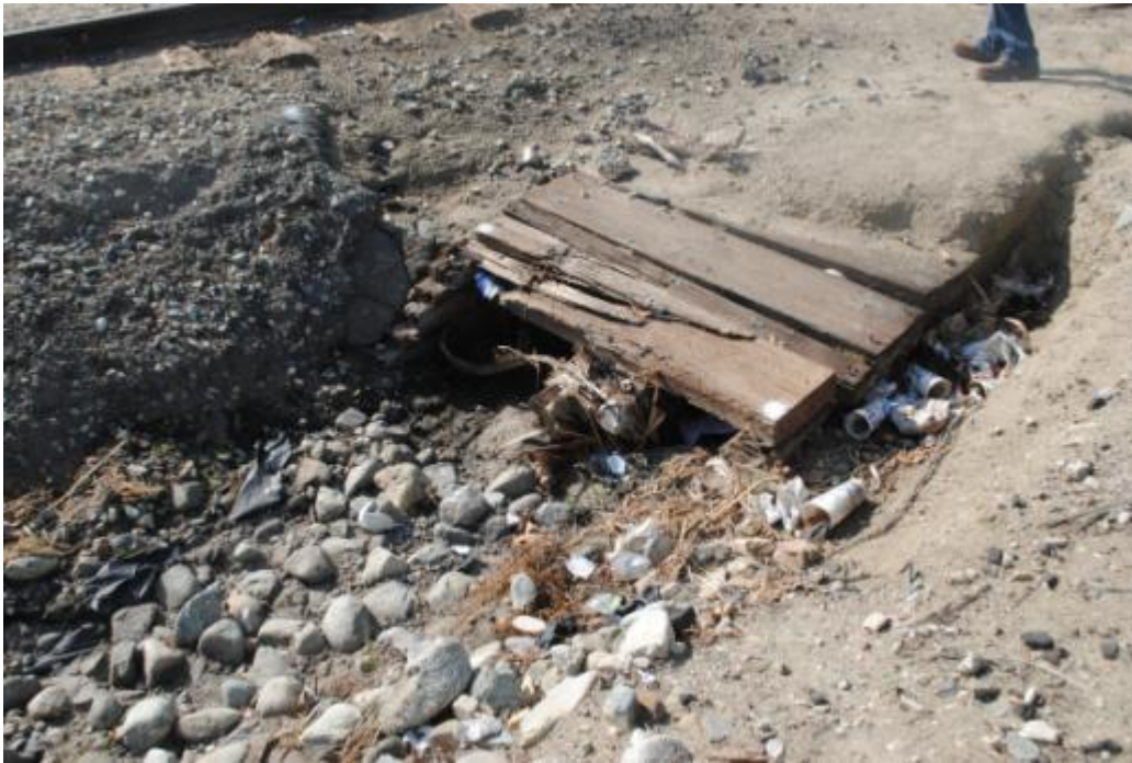
MP 7.4, 24-inch x 18-inch box culverts (no. 4)
