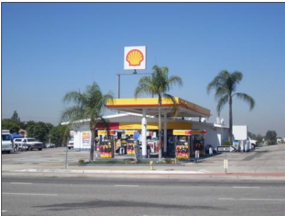
Photo 7: Shell Service Station with closed leaking underground storage tank (LUST) case onsite (Map Code U). View is toward the west.
