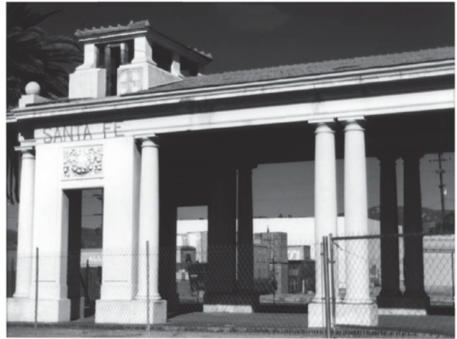
1991 photo. South elevation looking north
