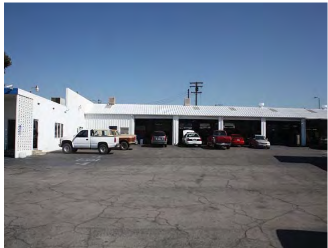
Looking east, rear elevation and attached building
