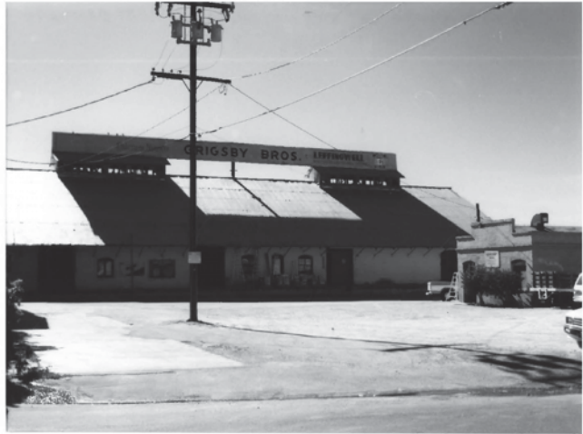
1991 photograph. North elevation looking southwest
