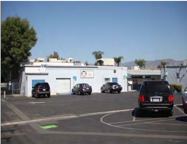
South elevation, looking north
