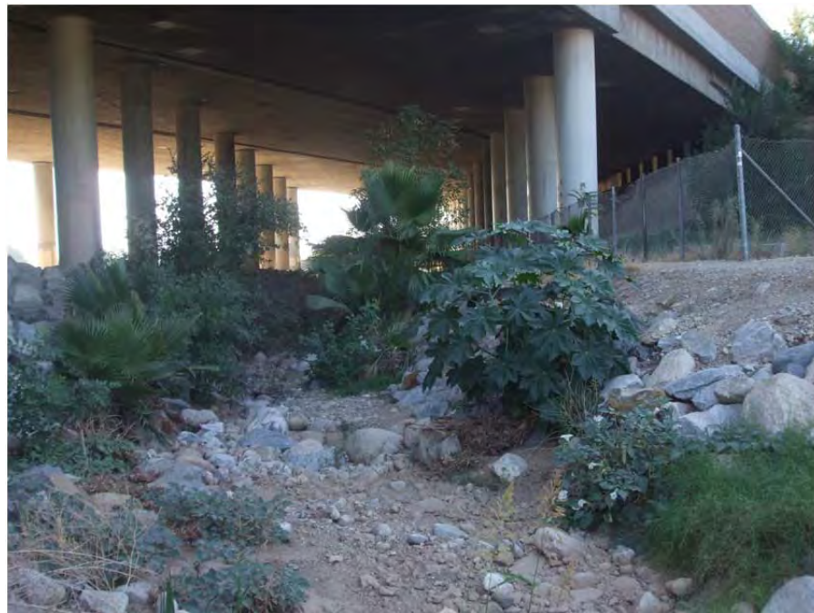
Photograph 4: Zanja underneath 1-10, view to west
