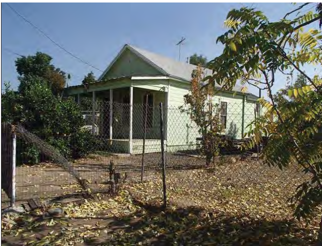
North and west elevations, looking southeast
