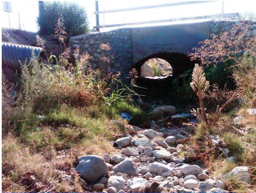
Photograph 7: Culvert at Church Street, note pipe at left, view to southwest
