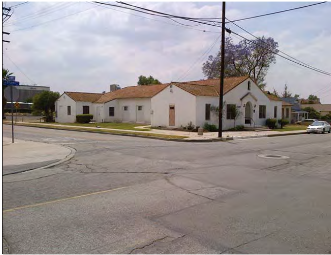
East and north elevations, looking southwest
