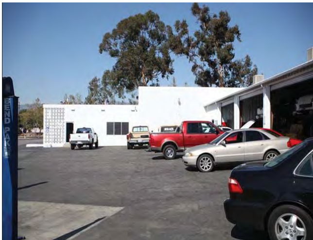
Looking north, rear elevation and attached building
