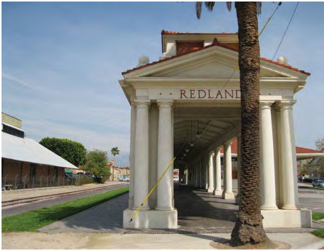
West elevation looking east
