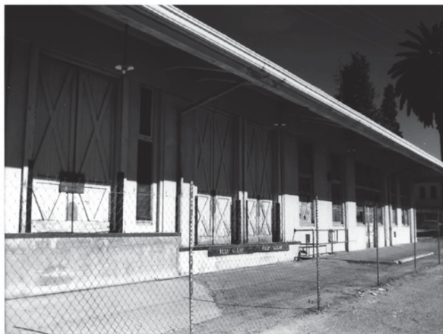
1991 photo. South elevation looking northeast
