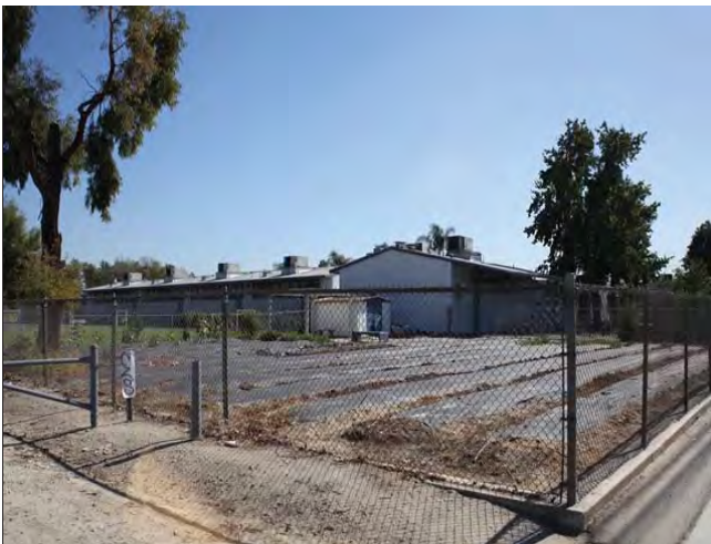
North elevation, looking southeast
