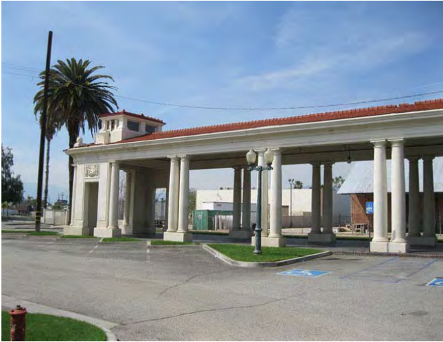
South elevation looking northwest
