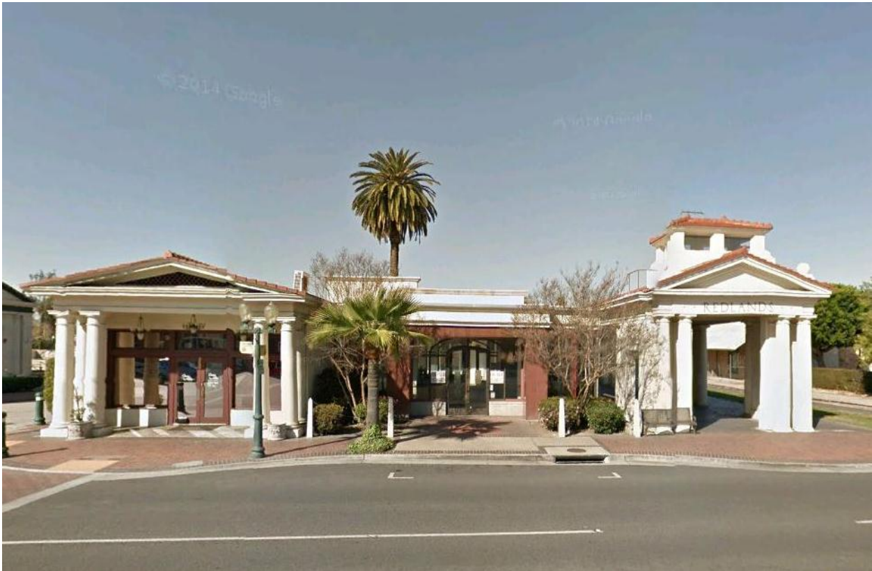
Figure 5-4. Redlands Santa Fe Station Today.
