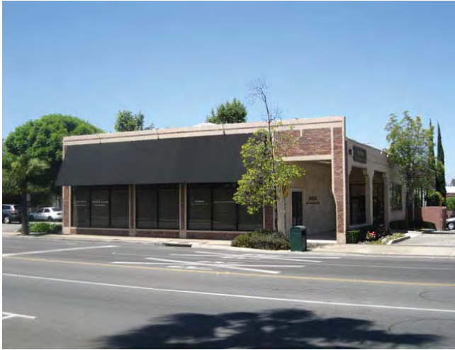
East and north elevations lkg southwest
