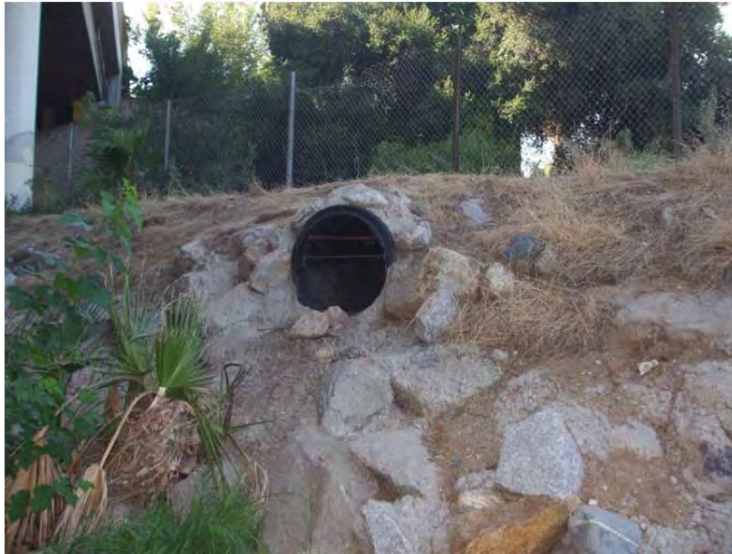
Photograph 3: Drainage pipe at north Zanja incline east of 1-10, view to north
