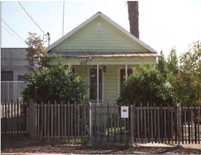
North elevation, looking south
