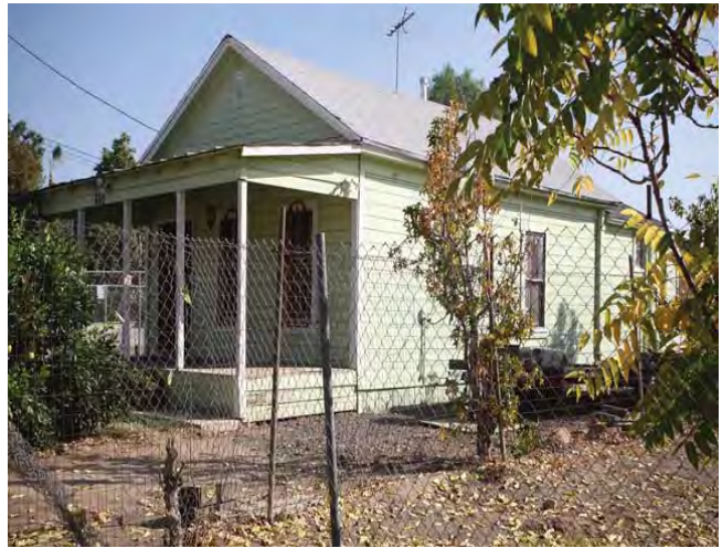
North and west elevations, looking southeast
