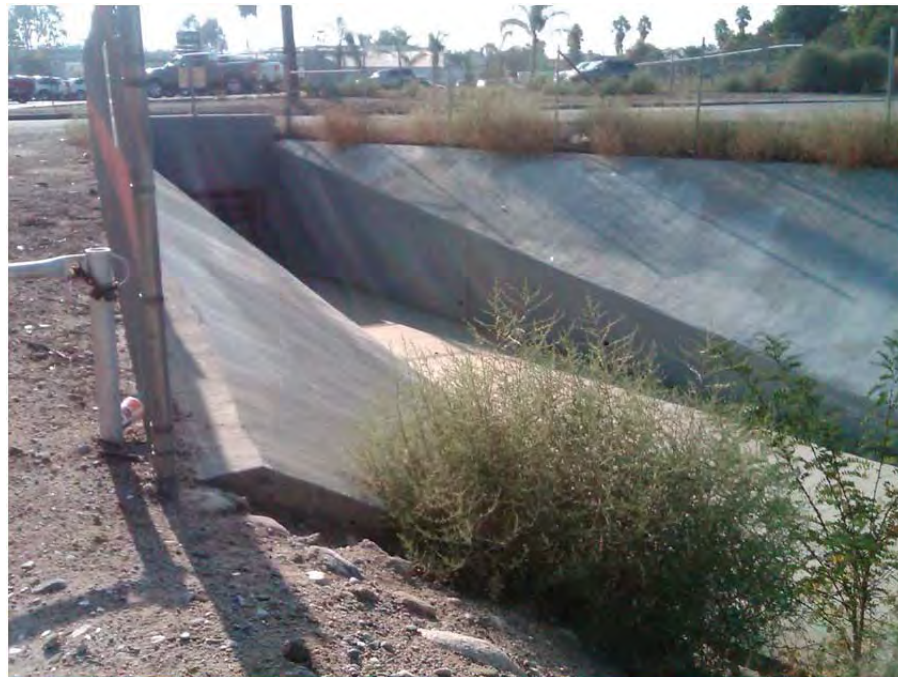
Photograph 9: Concrete channel portion of Zanja at 9th Street, view to northwest
