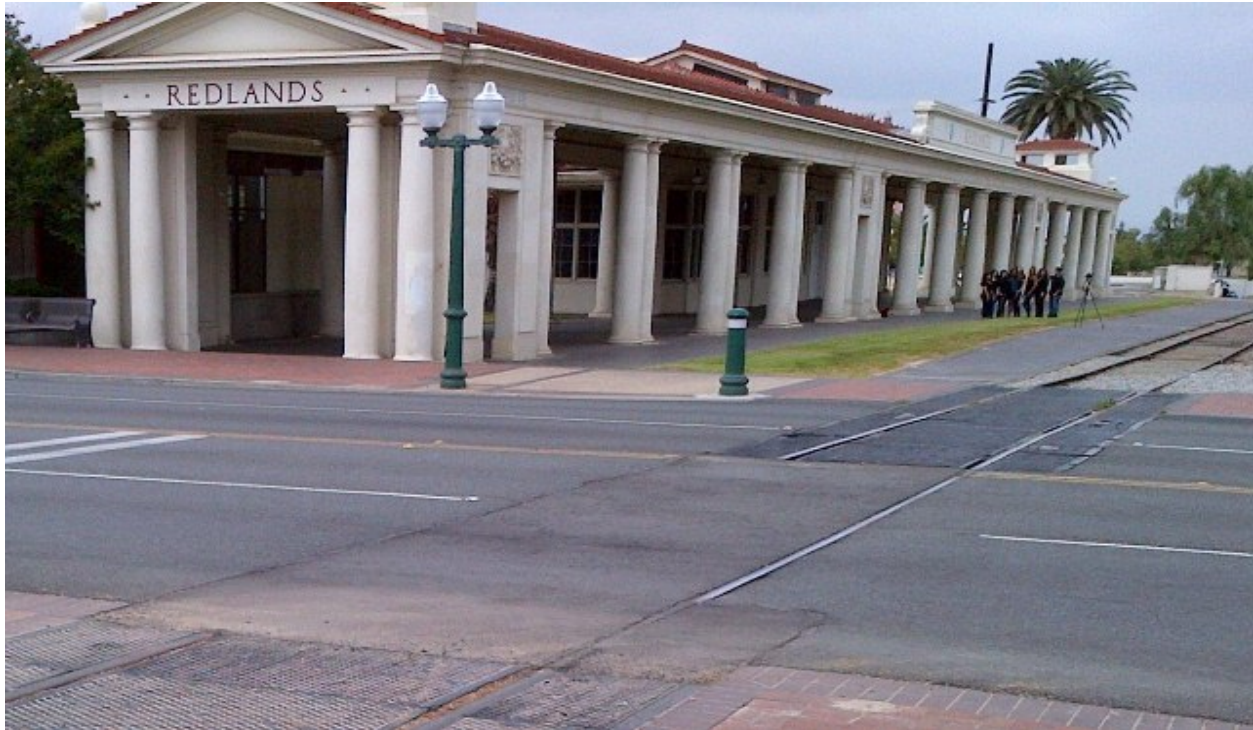
Figure 5-3. Redlands Santa Fe Station Today. View to west-southwest. Sidewalk, plaza, former spur track, and narrow landing area that would be altered under the Preferred Undertaking.
