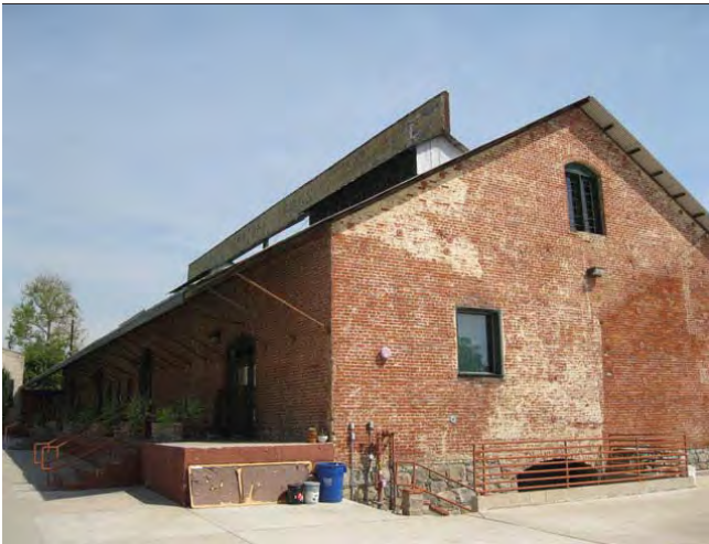
West and north elevations looking southeast
