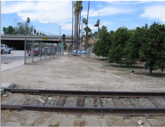
Looking north, California St on left, subject rail at bottom
