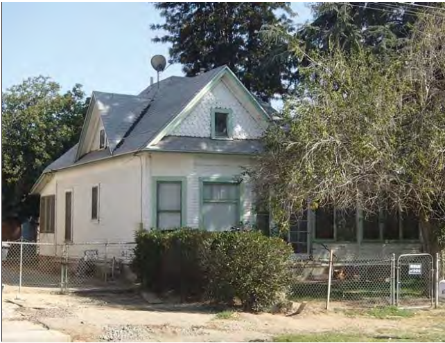
North and west elevations, looking southeast
