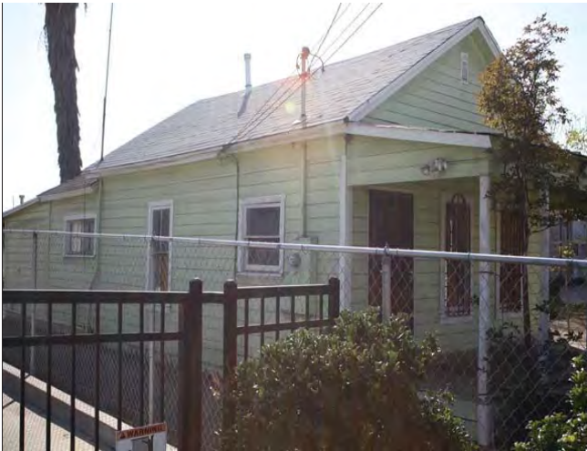
North and east elevations, looking southwest
