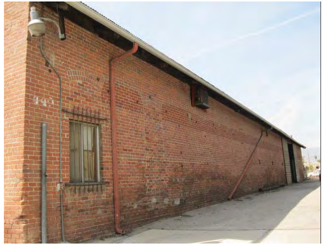
East elevation, looking northwest
