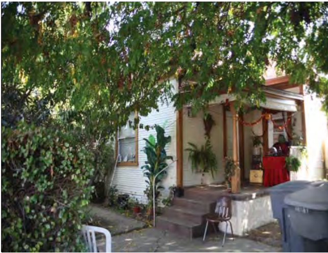
North and west elevations, looking southeast
