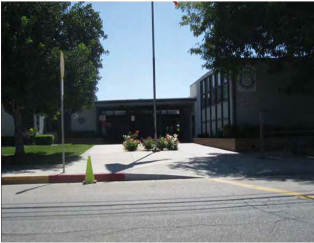
West elevation, looking east
