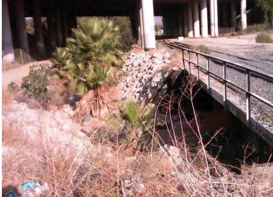
Photograph 5: Railroad bridge and riprap west of I-10, view to east
