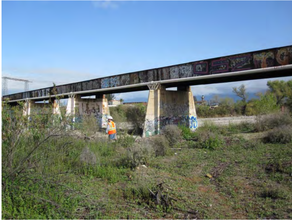
Figure 1: Santa Ana River, AT&SF Bridge 3.4 Downstream Face
