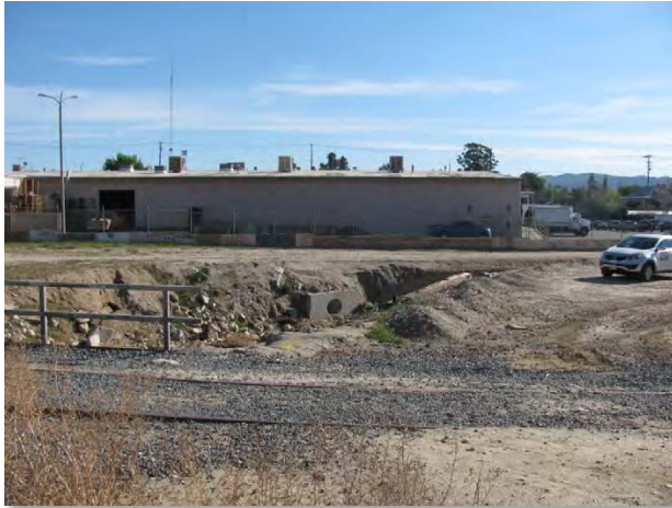
Photograph 1. Mill Creek Zanja. View facing south with Bridge 9.4 in foreground.
