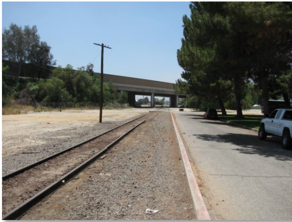
Photograph 3. Proposed basin site is located left of the tracks. View facing west toward I-10 overpass and Bridge 9.4.
