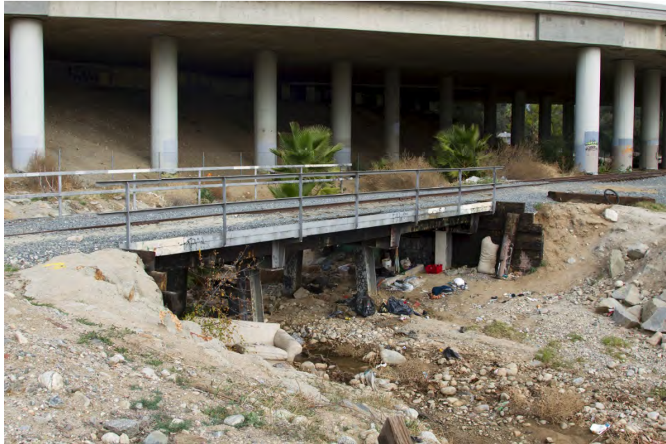
Figure 1: Bridge 9.4 Downstream Face
