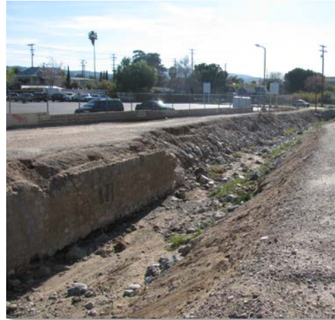
Photograph 2. Mill Creek Zanja. View facing southwest towards Church Street.
