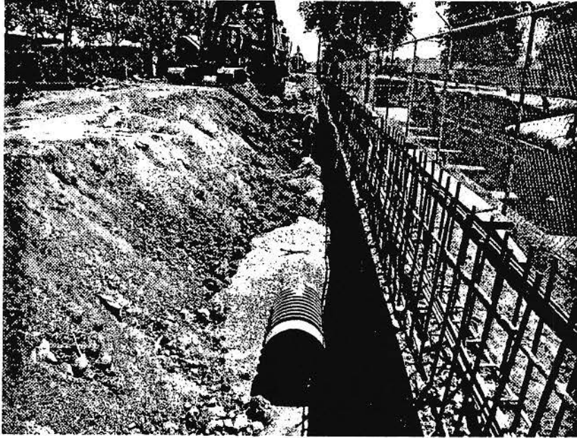
SOJV subcontractor Rainbow installing storm drain pipe near Balboa Blvd.
