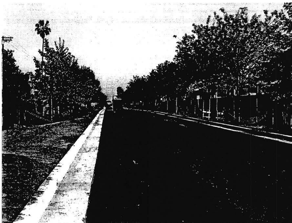
Paving operation along Chandler Boulevard.
