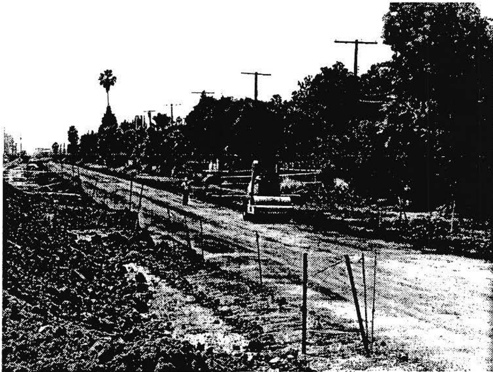
Placement of crushed miscellaneous base material.
