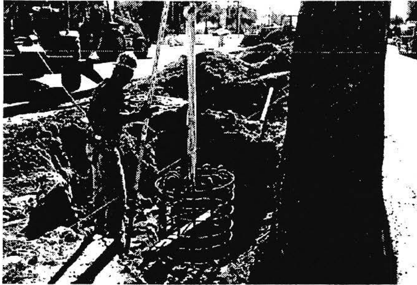
Installation of the cast in drilled hole piling system at Laurel Canyon Station
