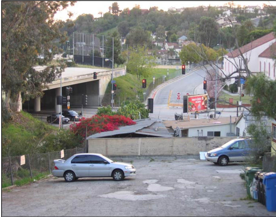
Figure 2-10. View Southwest of the SR-2 Terminus from Residential Areas to the East
