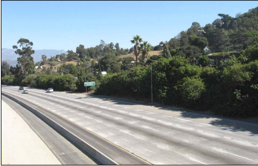
Figure 2-12. View Northeast along SR-2, from Oak Glen Place Overpass
