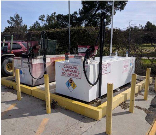
Photograph 3 – Adjoining Property – Golf Course Bldg.
