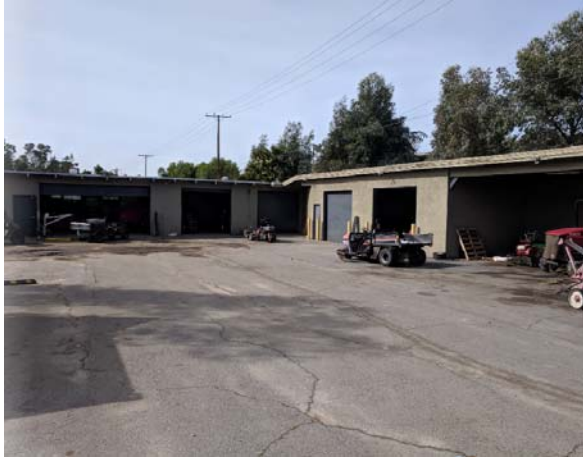
Photograph 1 - Adjoining Property – Golf Course Bldg.
