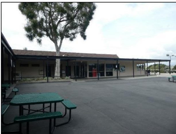
Figure 9. View of the east elevation of the western section, view facing west. Note the projecting rectangular mass on this elevation. Source: GPA Consulting 2019.
