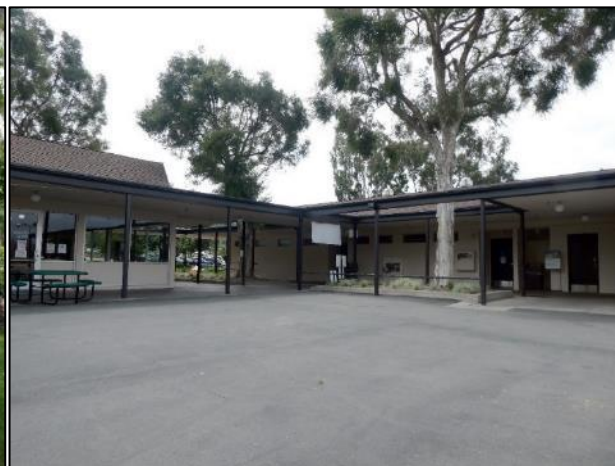
Figure 7. View of the courtyard formed by the eastern section and western section, view facing southwest. Note the covered breezeway and walkways that unite both sections of the building. Source: GPA Consulting 2019.
