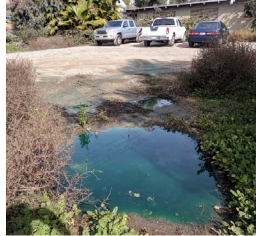
Photograph 2 - Adjoining Property – Golf Course Bldg.
