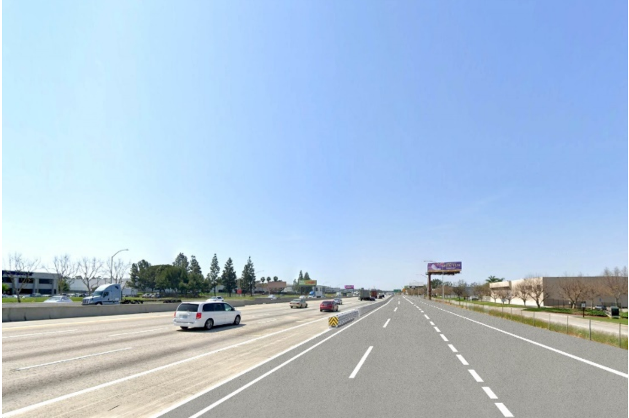
Figure 2.6-4. Key View 2 – Visual Simulation of Proposed Improvements (Eastbound and westbound SR-91 is widened with new concrete barriers, and a retaining wall is constructed on the eastbound side)
