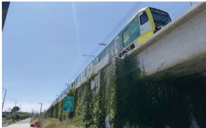
Aerial Guideway Transition to At-Grade Level over Retaining Wall on the Metro E Line
