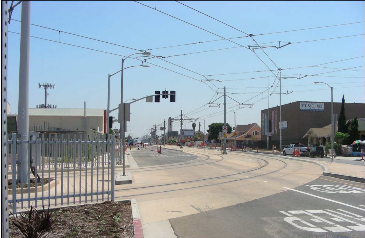
Figure 2.13. Example of At-Grade Guideway with Embedded Trackwork through Intersection on Existing Eastside Line
