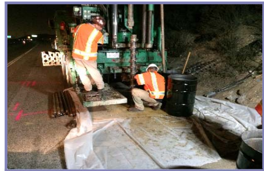
Drilling for a Soil Boring
