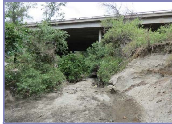
SR 60 Freeway Crossing over Rio Hondo
