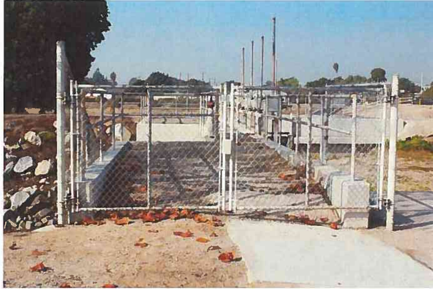
Photograph 6. Paved Surface on Top of Gate (nonfunctional), View to West
