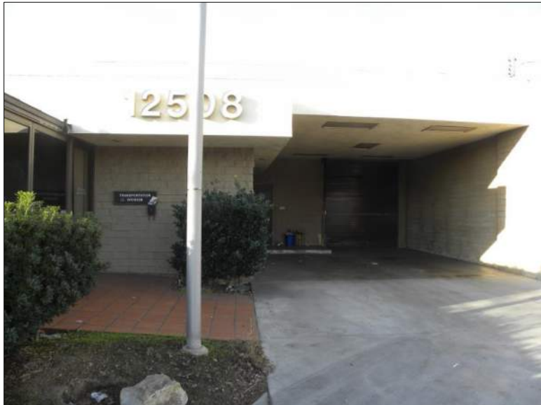
Photograph 2. View of E elevation, camera facing west, 12/17/2019, DSCN0122
