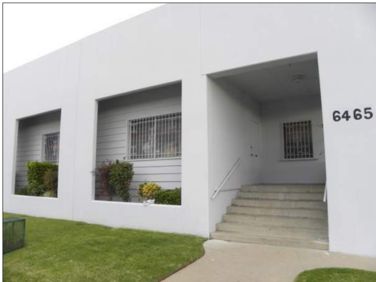
Photograph 2. View of S elevation/façade, camera facing north, 12/18/2019, DSCN0262
