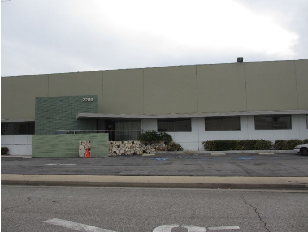
Figure 6.12. Former Sues, Young & Brown Inc. Building constructed 1956 (2200 Saybrook Avenue) View Southeast
