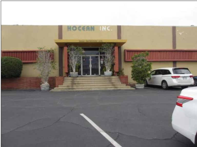
Photograph 2. View of south elevation, camera facing north, 12/18/2019, IMG_9233
