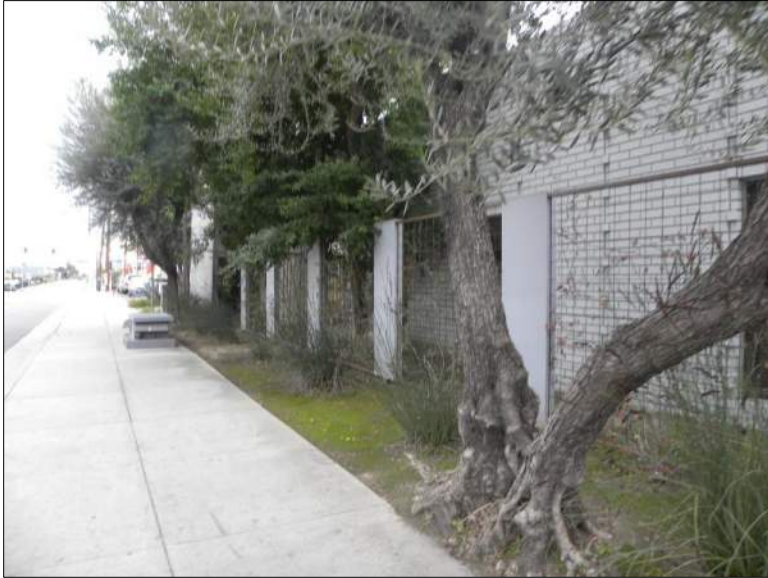
Photograph 2. View of N elevation, camera facing southeast, 12/18/2019, DSCN0292
