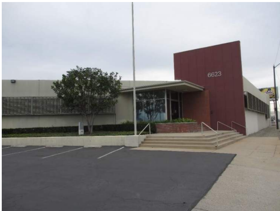
Photograph 5. Former Hoffman Hardware Company building (6625 E Washington Boulevard), view north
