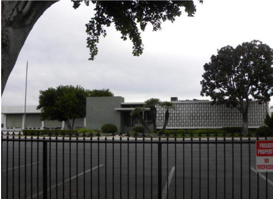
Photograph 11. Property located at 6433 Gayhart Street, view northeast
