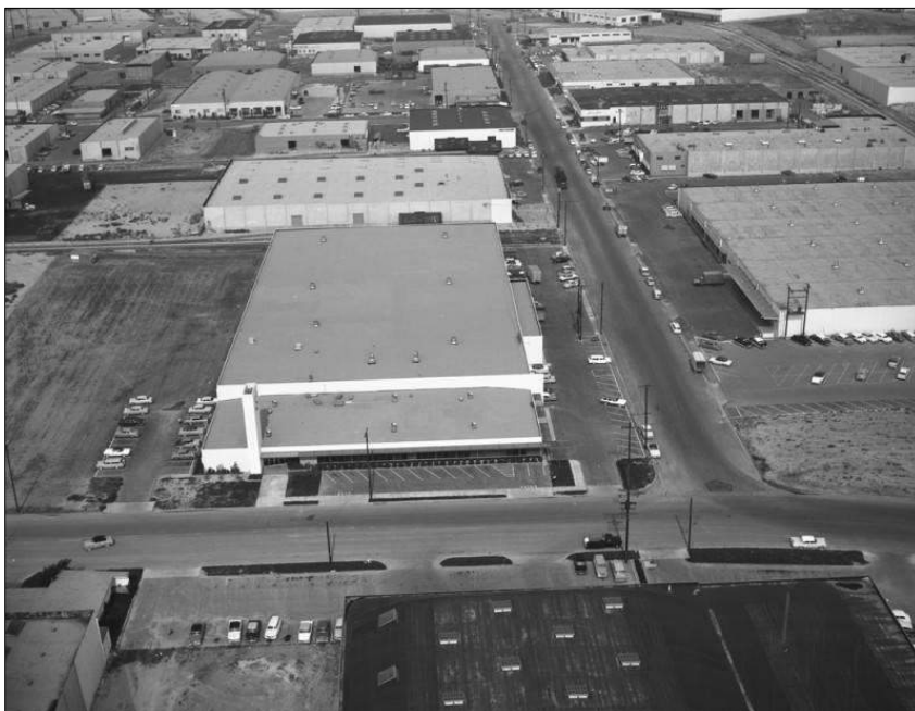
Plate 12. Sylvania Electric Products building (6505 Gayhart Street), view to north, 1957 (LAPL 1957).
