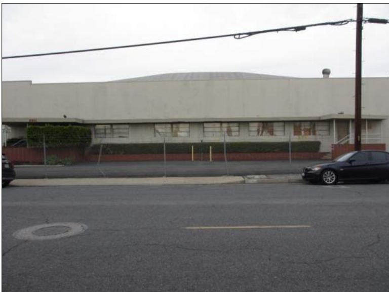
Photograph 2. View of west elevation, camera facing east, 12/18/2019, IMG_9221
