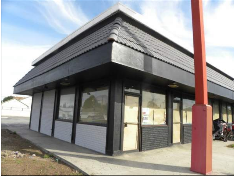
Photograph 2. View of South and east elevations, camera facing west, 12/17/2019, DSCN0151
