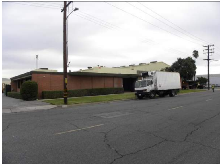
Photograph 4. View of SW elevation/façade, camera facing NE, 12/18/2019.
