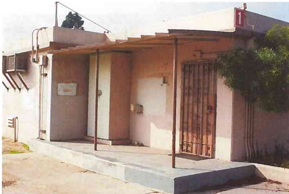
Photograph 7. Control Station Structure, View to Southwest
