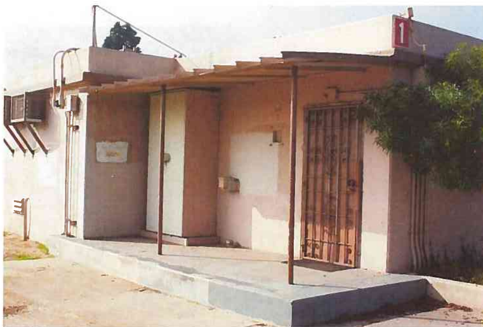
Photograph 7. Control Station Structure, View to Southwest
