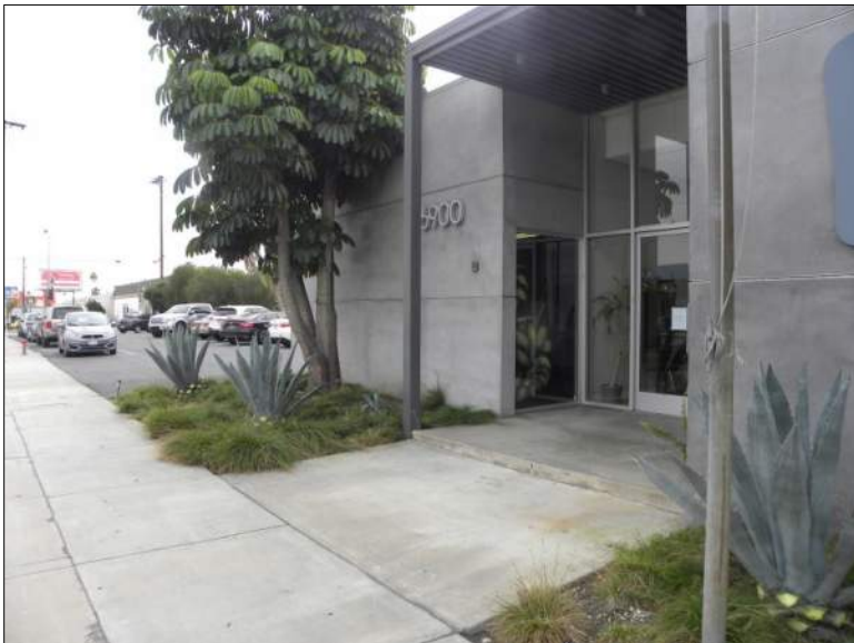
Photograph 3. View of entry, camera facing southeast, 12/18/2019, DSCN0293
