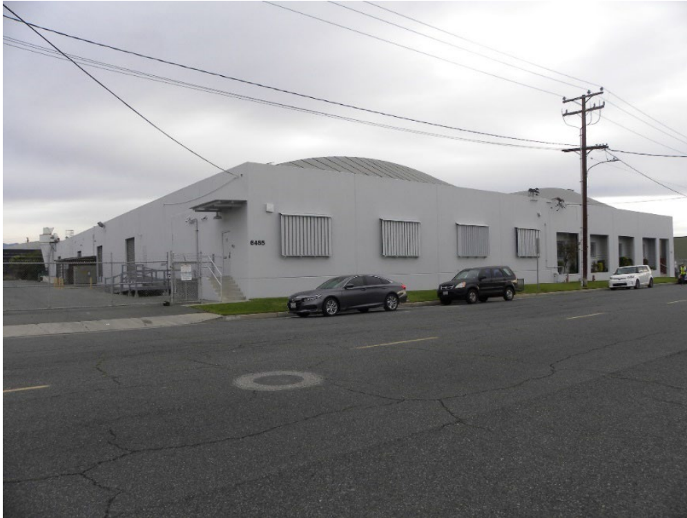
Figure 6.8. Former Titanium Metals Corporation of America Building constructed 1954 (6465 Corvette Street) View East
