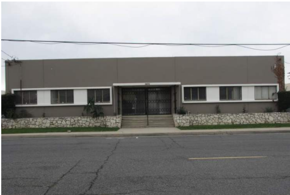
Photograph 12. Property located at 6436 Corvette Street, view southwest
