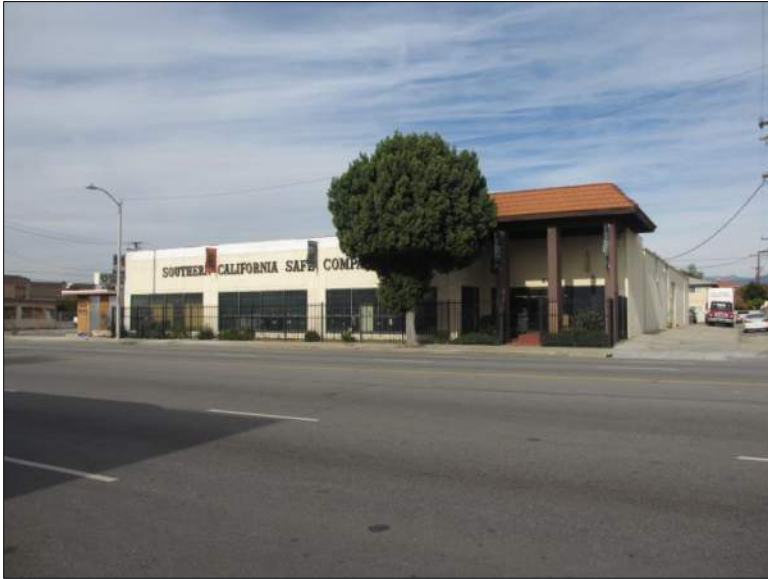
Photograph 2. View of S elevation, camera facing east, 12/17/2019, IMG_9129
