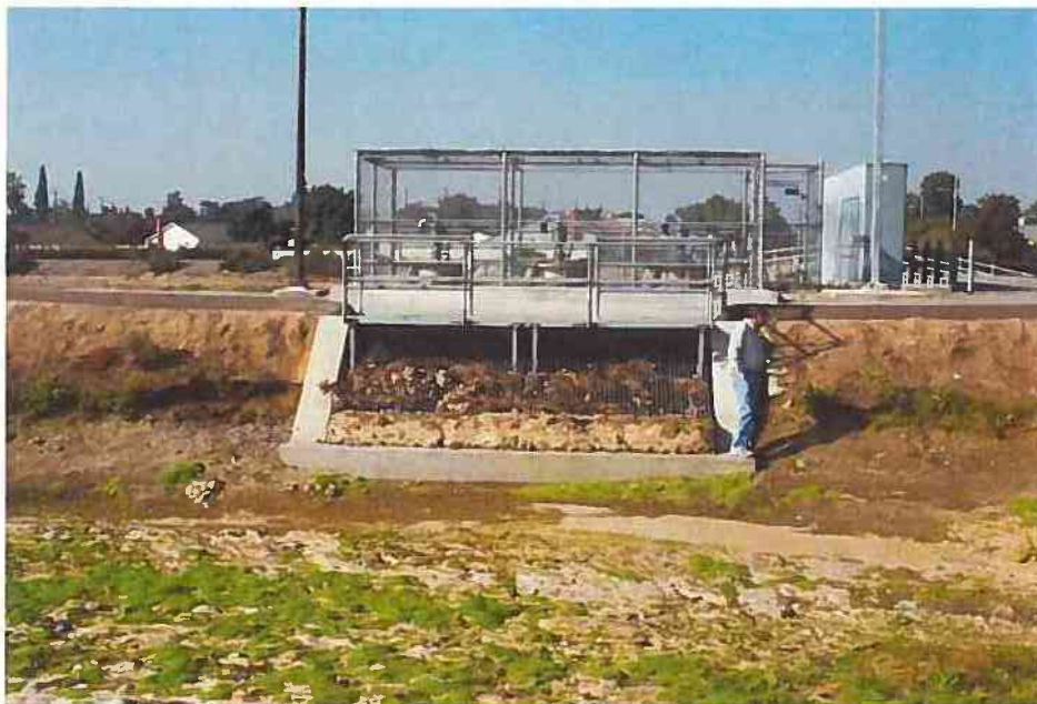
Photograph 10. Mine Avenue Pump Station, View to West
