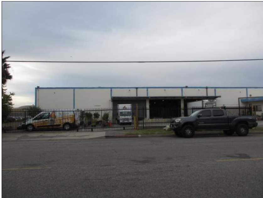
Photograph 2. View of NE elevation loading docks, camera facing west, 12/18/2019, IMG_9167
