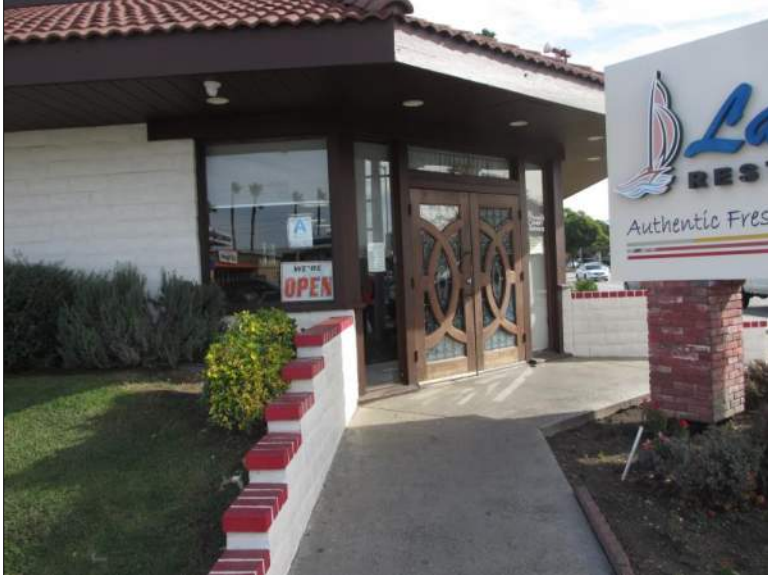
Photograph 2. View of entrance, camera facing east, 12/17/2019, IMG_9126
