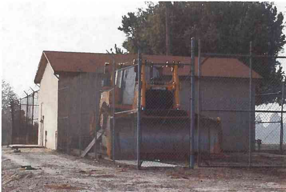
Photograph 9. Control Station Shed 2, View to Southwest
