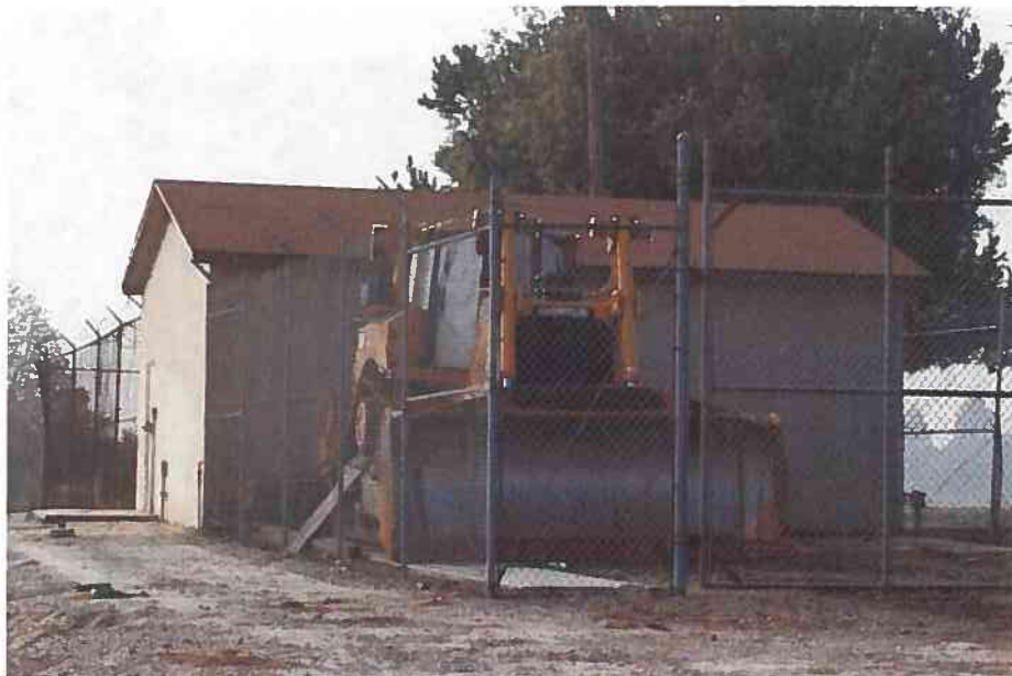
Photograph 9. Control Station Shed 2, View to Southwest
