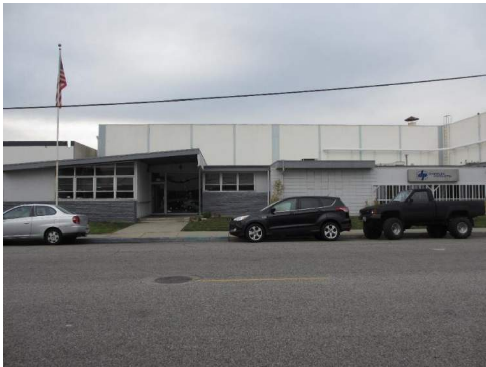
Photograph 4. Former Marwais Steel Company building (6466 Gayhart Street), view southwest
