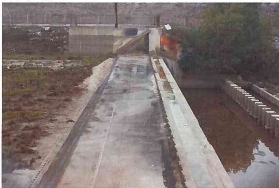
Photograph 11. Rubber Dam No. 2, View to East
