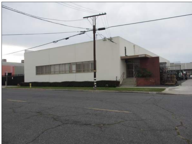
Photograph 2. View of N elevation/façade, camera facing SE, 12/18/2019.
