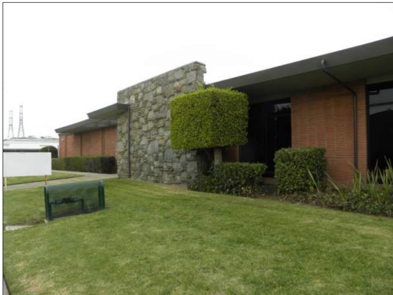
Photograph 2. View of S elevation/façade, camera facing NW, 12/18/2019.
