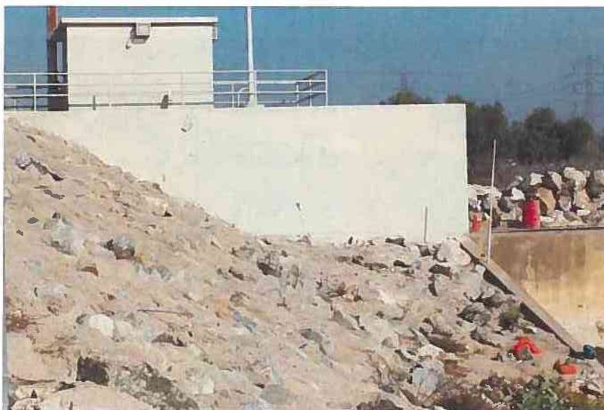
Photograph 13. Control Station for Rubber Dam No. 4, View to Northeast
