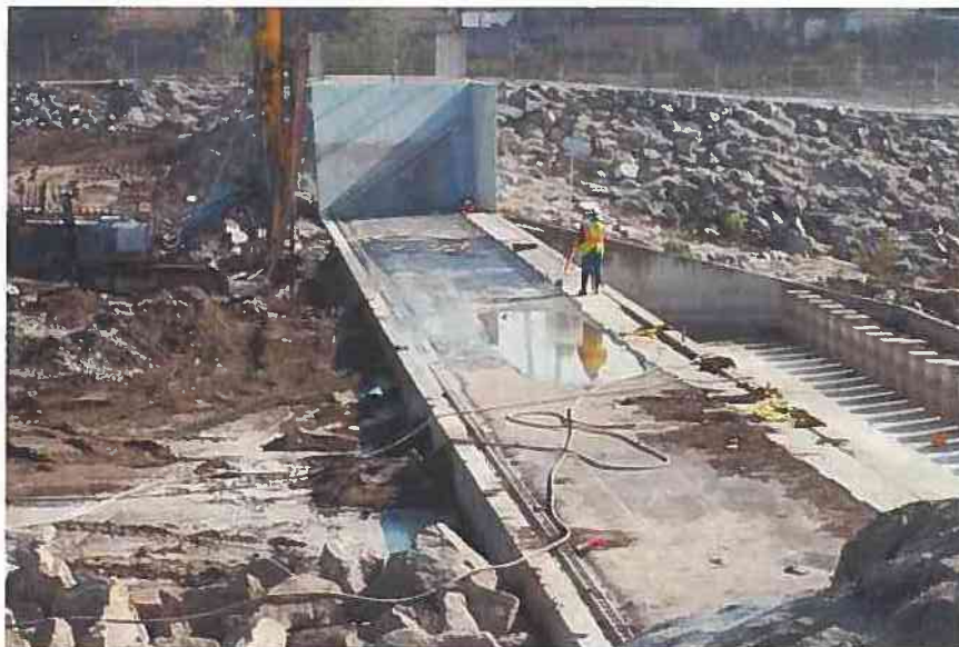
Photograph 12. Rubber Dam No. 4, View to Southeast
