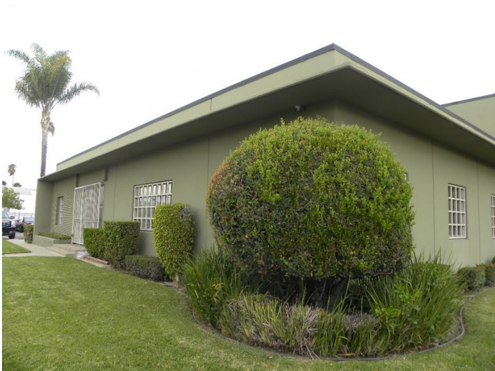
Figure 6.7. Former Bralco Metals Company Building constructed 1954 (6489 Corvette Street) View Northeast
