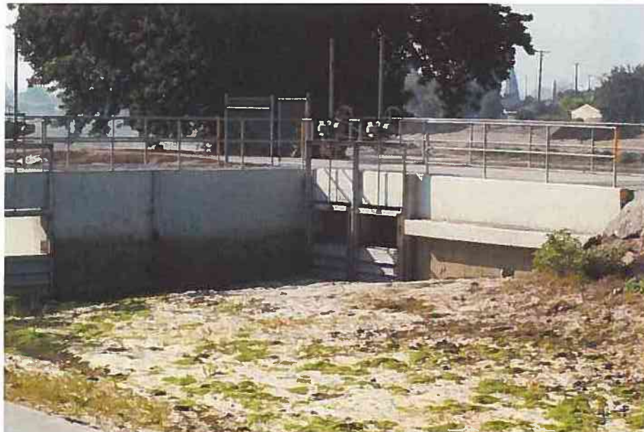
Photograph 5, Gate #2, View to Southwest
