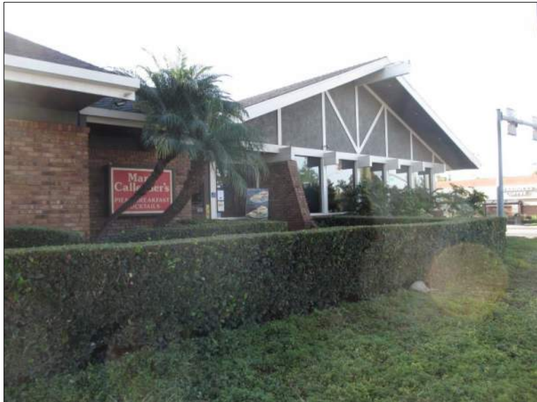
Photograph 2. View of N elevation, camera facing south, 12/17/2019, IMG_9096
