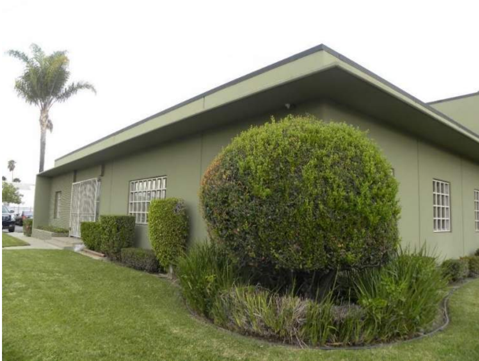
Photograph 1. Former Bralco Metals Company building (6489 Corvette Street), view northeast
