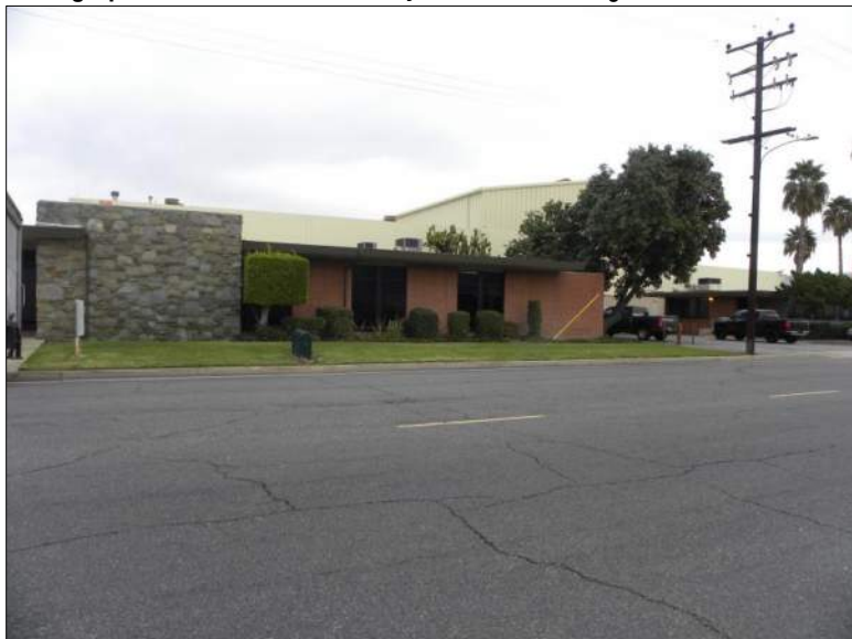
Photograph 3. View of S elevation/façade, camera facing N, 12/18/2019.
