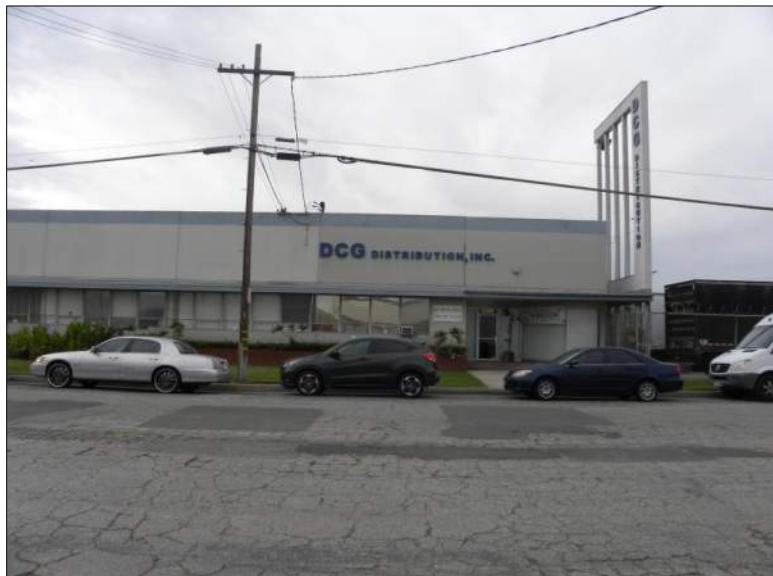
Photograph 2. View of E elevation, camera facing west, 12/18/2019, DSCN0279
