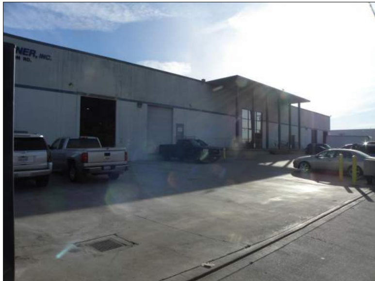
Photograph 2. View of SW elevation/façade, camera facing east, 12/17/2019, DSCN0128
