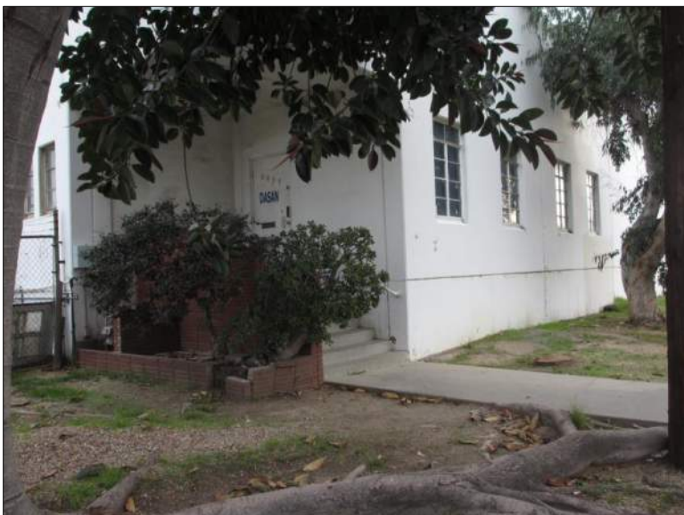
Photograph 2. View of entrance, camera facing SW, 12/18/2019, IMG_9187
