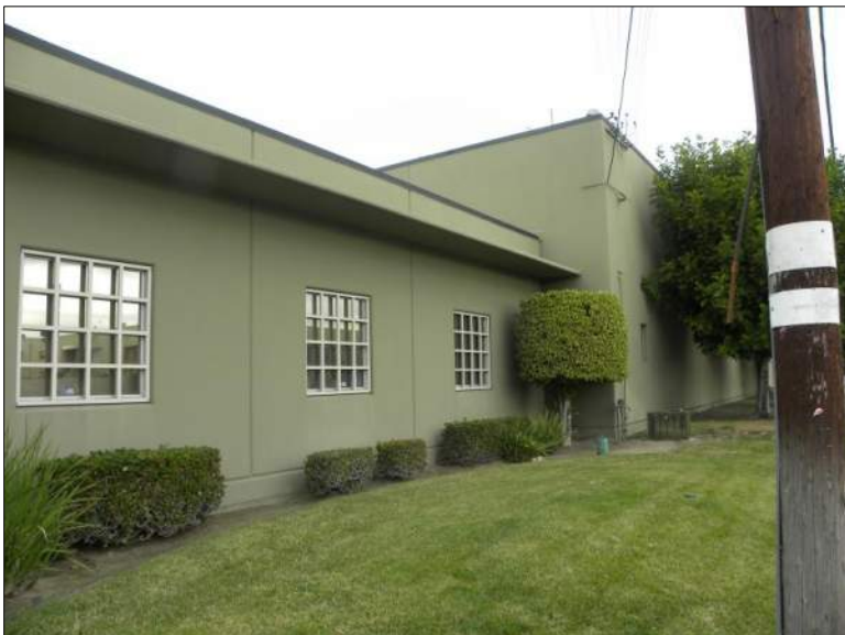
Photograph 2. View of E elevation/façade, camera facing north, 12/18/2019, DSCN0257
