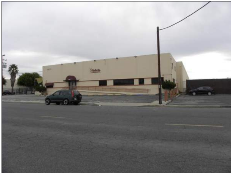
Photograph 2. View of east and south elevations, camera facing west, 12/18/2019, DSCN0272
