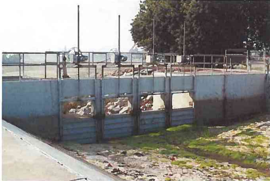
Photograph 4, Gate # 1, View to Southwest
