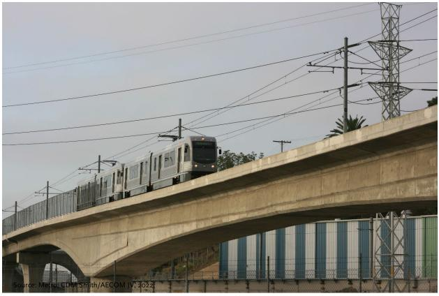
Figure 3.5. Example of an Aerial Structure
