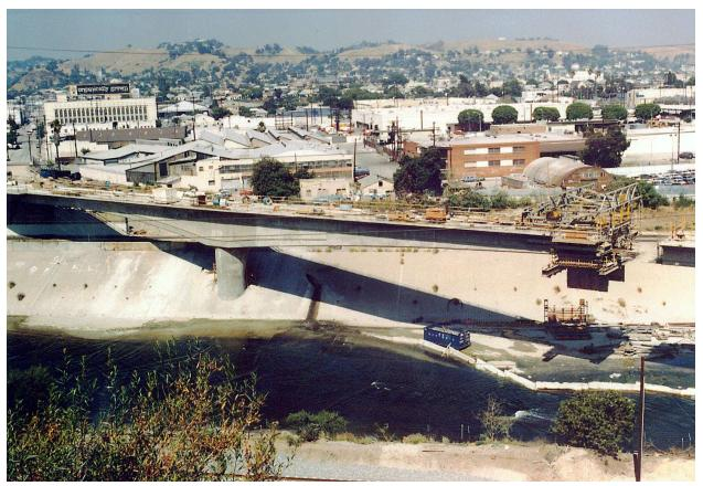
Source: Metro; CDM Smith/AECOM JV, 2019. Figure 3.8. Example of LRT Bridge Construction over a Waterway over the Los Angeles River at Chinatown
