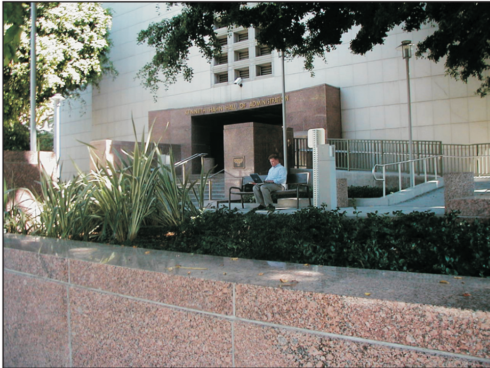
Photograph 2: Grand Avenue entrance to the Hall of Administration.
