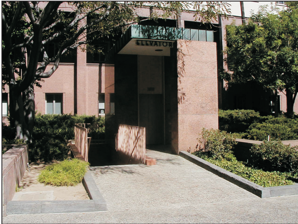
Photograph 2: Elevator located near south entrance of Hall of Administration
