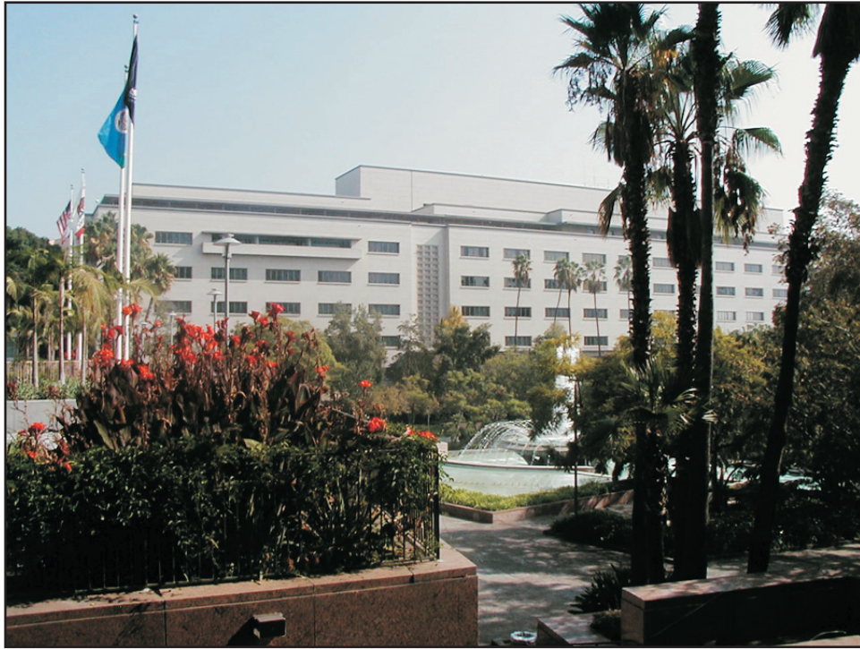
Photograph 1: Kenneth Hahn Hall of Administration, south elevation.
