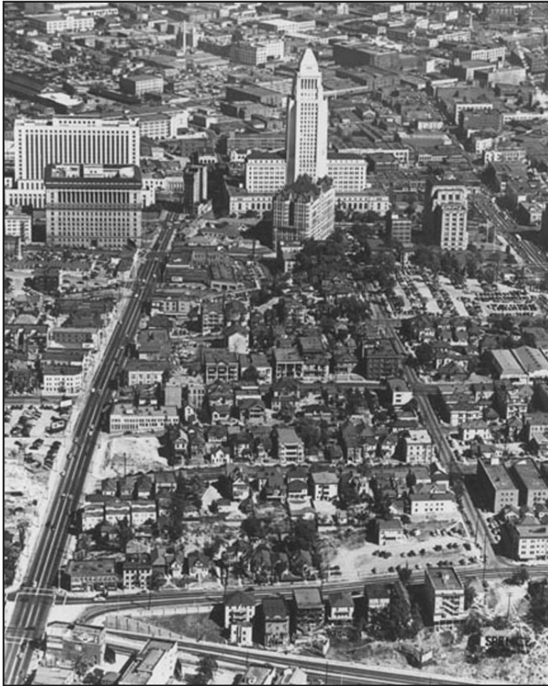
Photograph 1: Aerial view of City Hall and Bunker Hill circa 1940.
