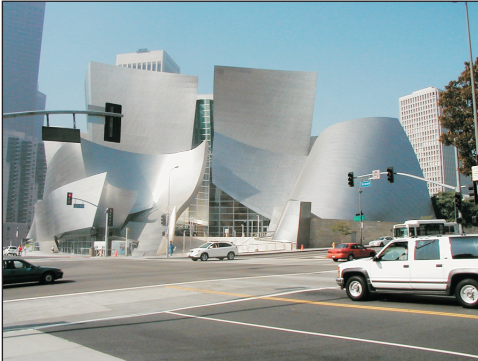
Photograph 1: Walt Disney Concert Hall at Grand Avenue and 1st Street.
