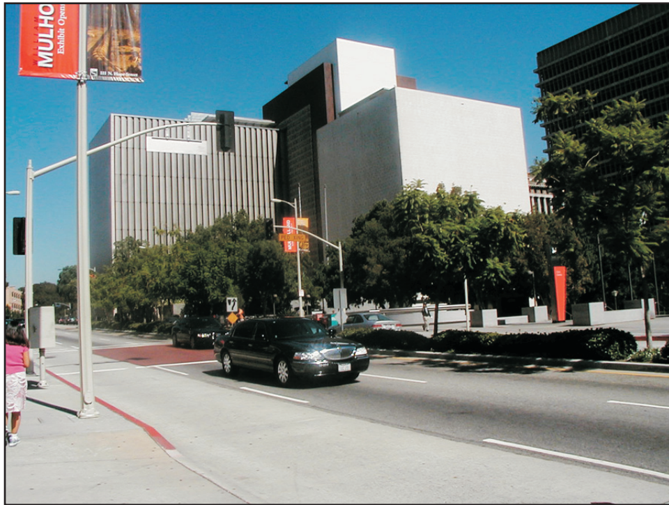
Photograph 1: Hall of Records south elevation.
