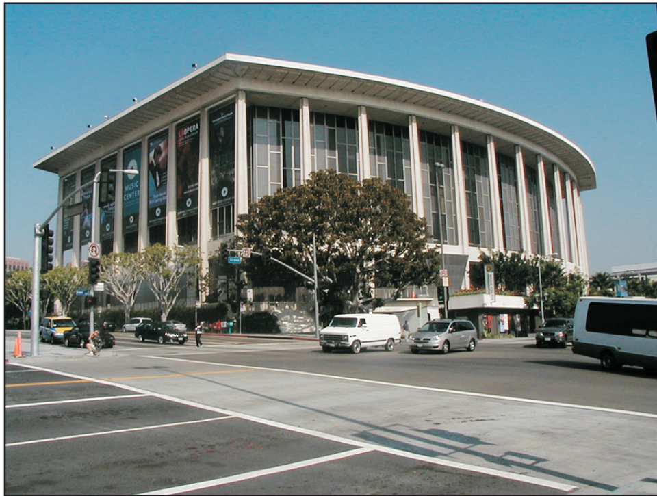
Photograph 1: Dorothy Chandler Pavilion at Grand Avenue and 1st Street.
