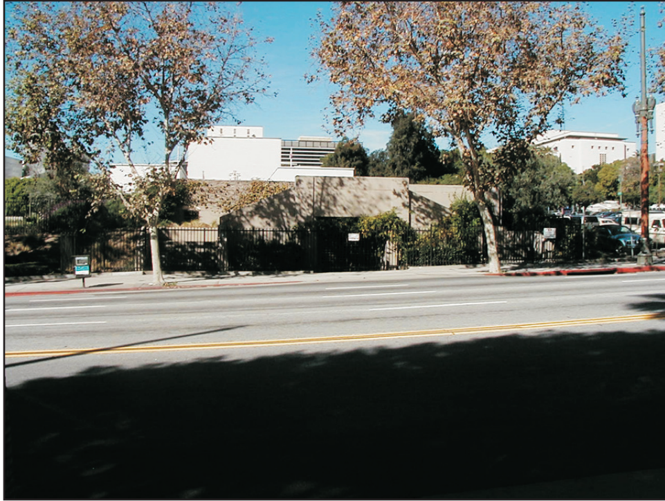
Photograph 1: Foundation of demolished State Office Building.
