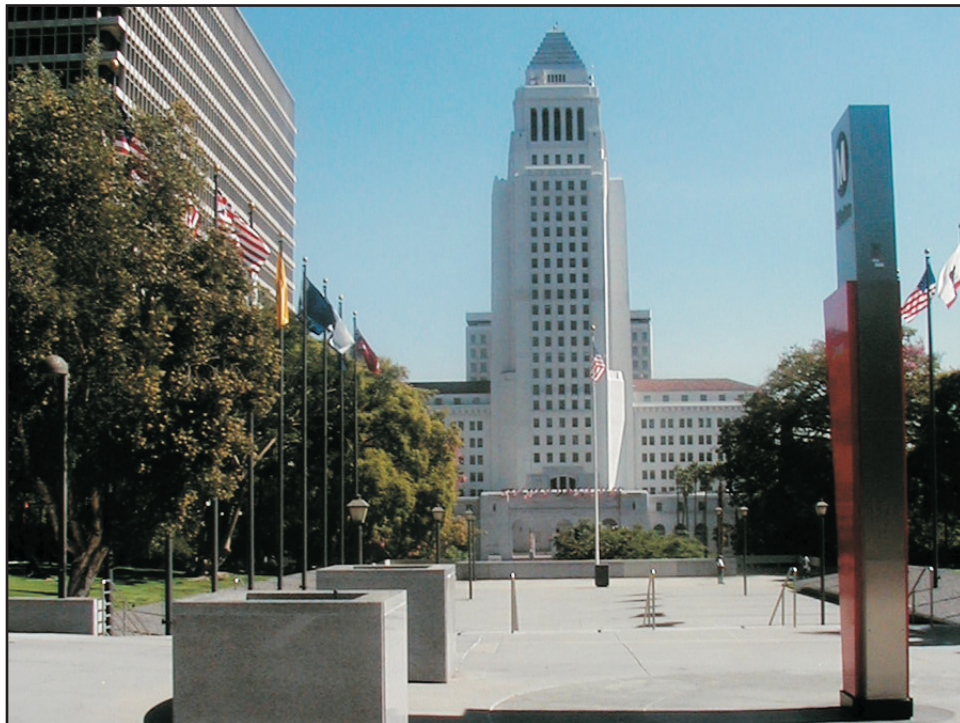
Photograph 2: Court of Flags looking east to City Hall.
