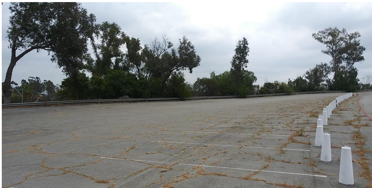
Photo 21. Southeast-facing view of proposed location for the Dodger Stadium Station in parking area. Site occurs in the paved area and roughly between tall trees at far left and right in photo.
