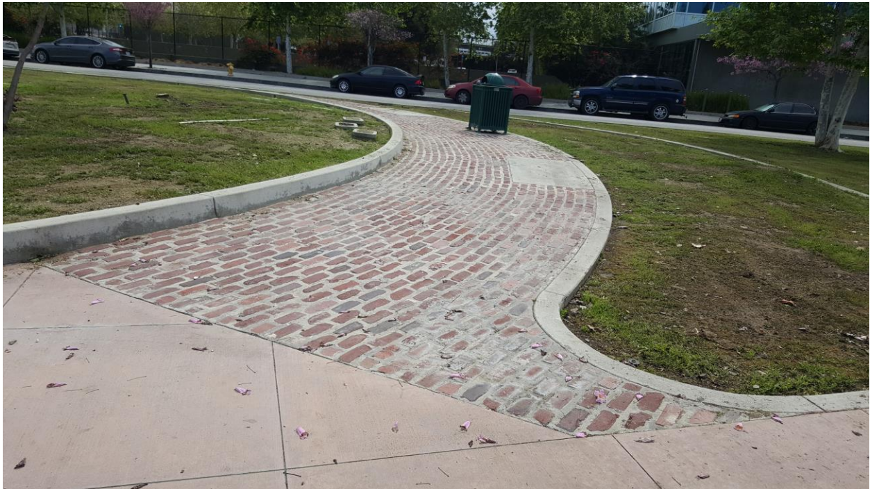
Plate 14: Brick Pavement Taken from Site 19-004200 and Reused Within 19-004201.
