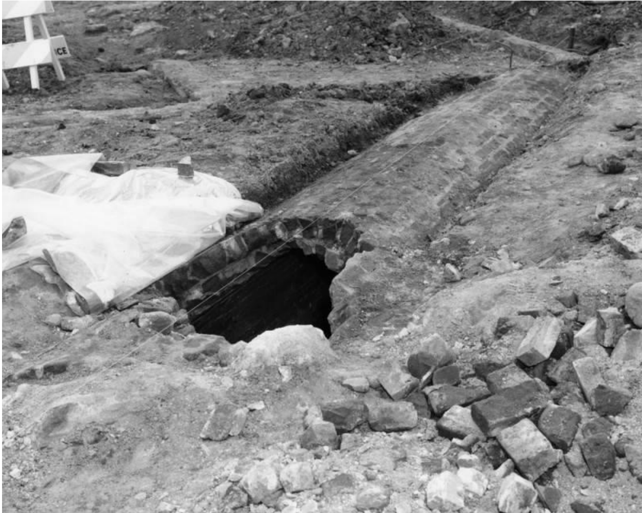
Plate 3: Zanja Madre segment excavated within La Placita de Dolores (19-000887) in 1978 (Security Pacific National Bank Photo Collection. Los Angeles Public Library 1978).
