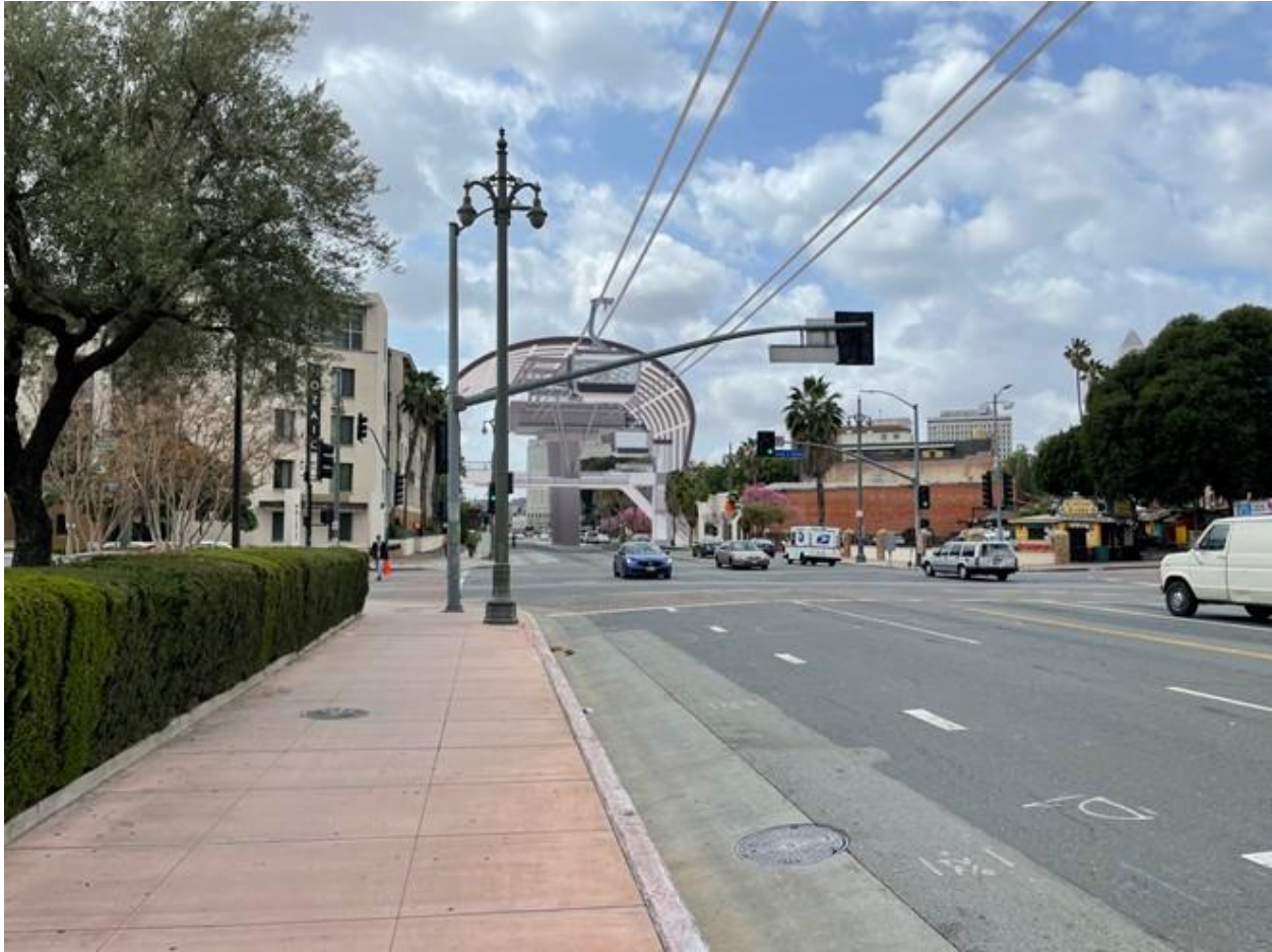
Figure 43: View of Alameda Station looking south on Alameda Street from just north of Cesar E. Chavez Avenue. RIOS, 2021.
