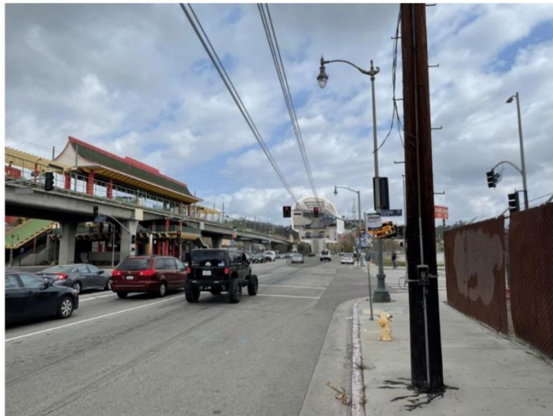
Figure 5-13: Existing and Simulation Views of KOP 12 – Looking North on Alameda Street/Spring Street from South of College Street
