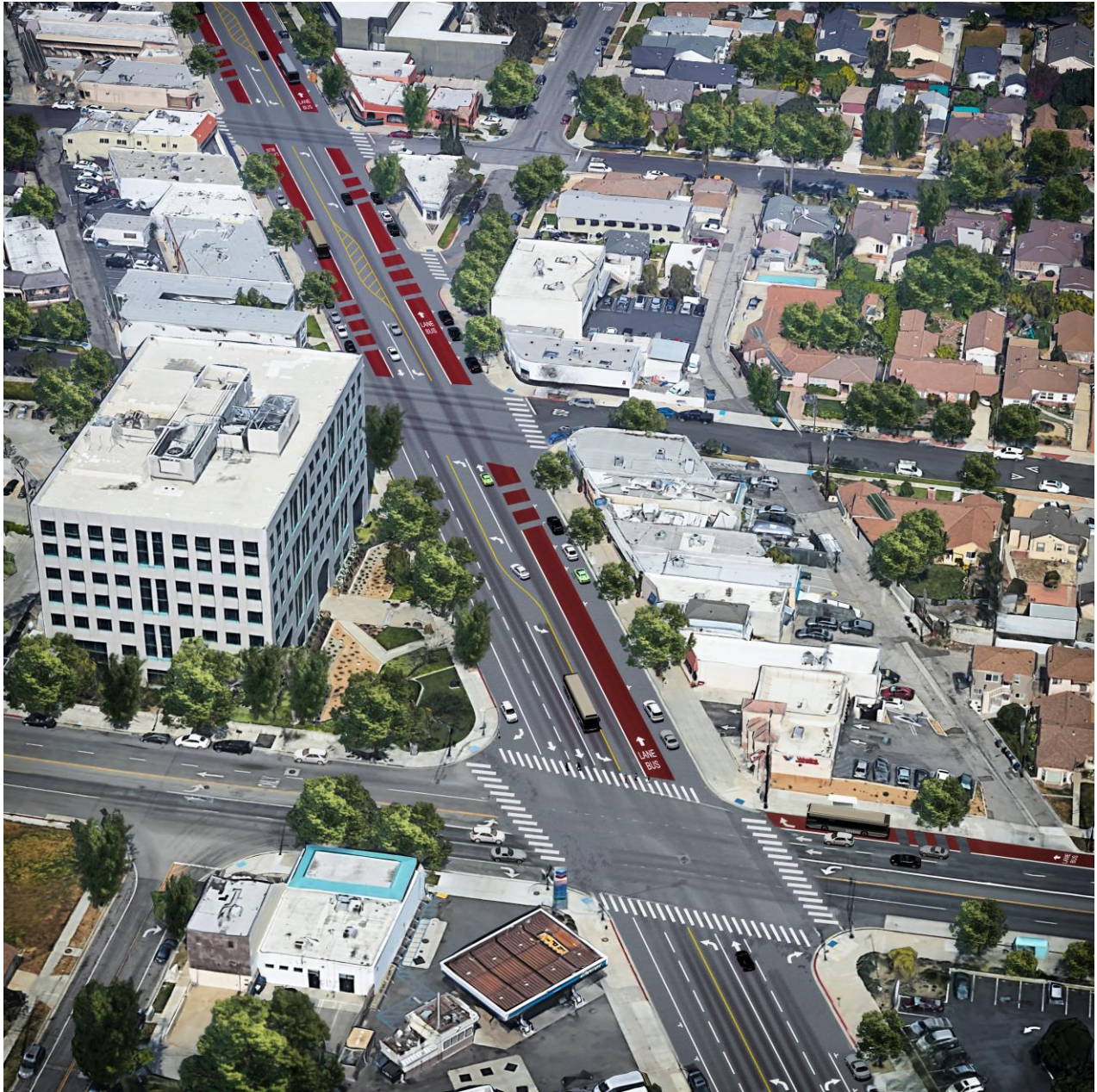
Figure ES-6 – Burbank – Olive Avenue Post-Project
