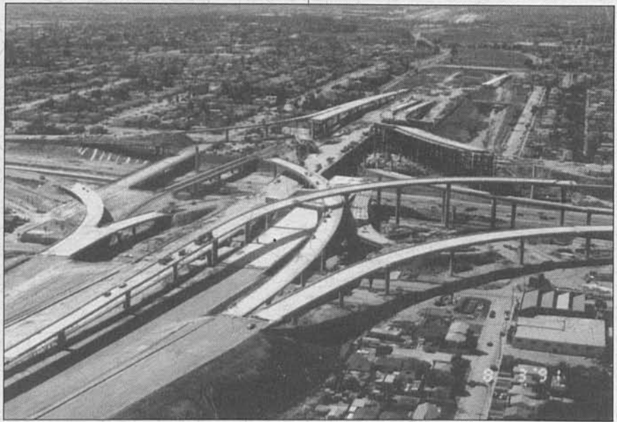
A view from above of the I-110/I-105 interchange. The Metro Green Line stations will be between the east and westbound structures of the I-105, where the Green Line will travel down the freeway median.
