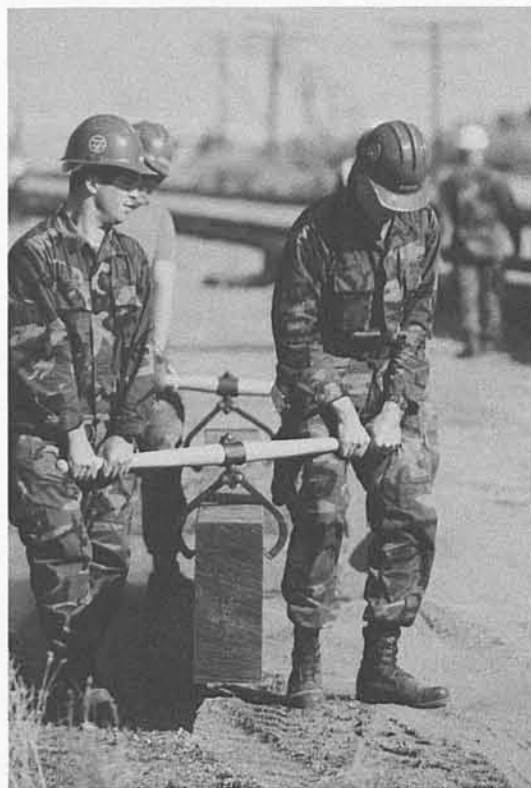
Navy Seabees working on tracks.
