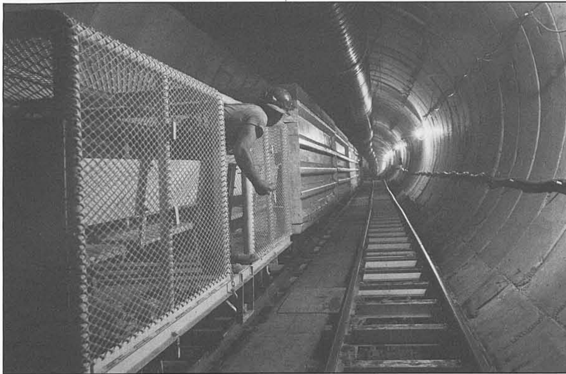
Metro Rail worker inside a Segment 2 Red Line Tunnel under construction.
