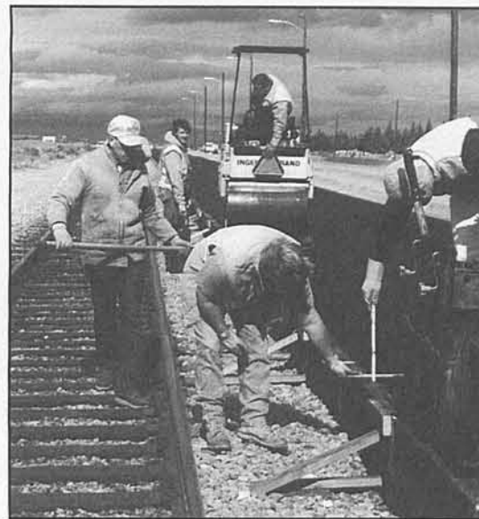
Workers maintain Metrolink tracks.
