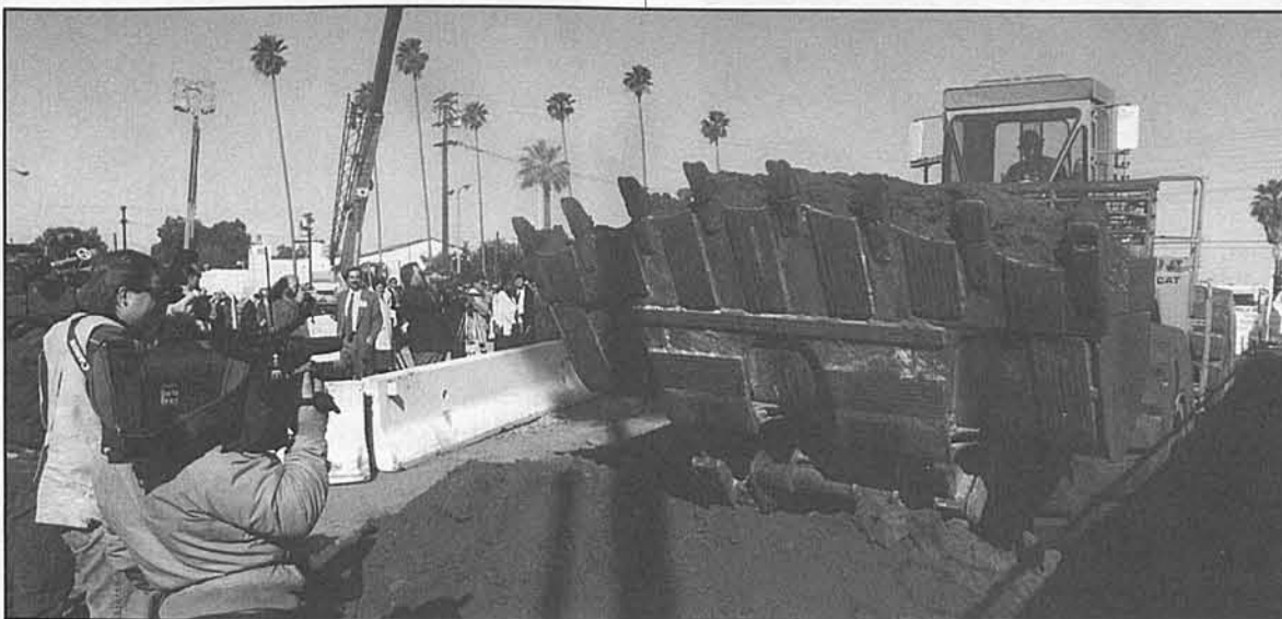
Television crews record the first shovelful of dirt turned for Segment 3.
