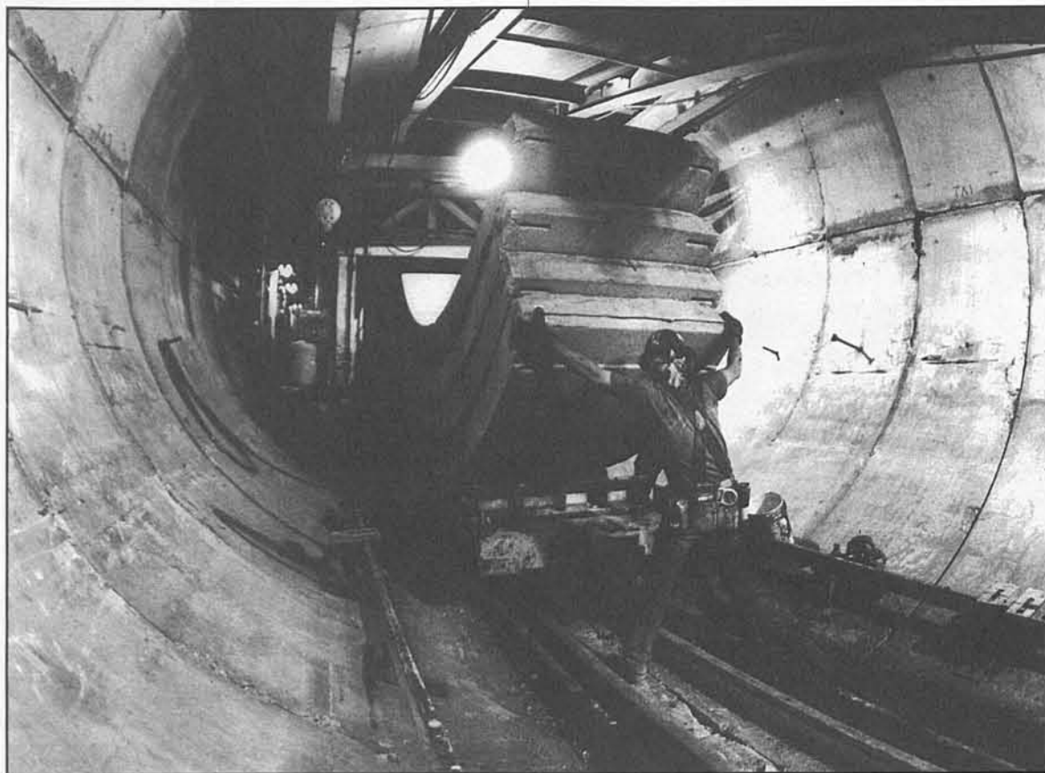
A tunnel builder readies concrete tunnel sections for installation.
