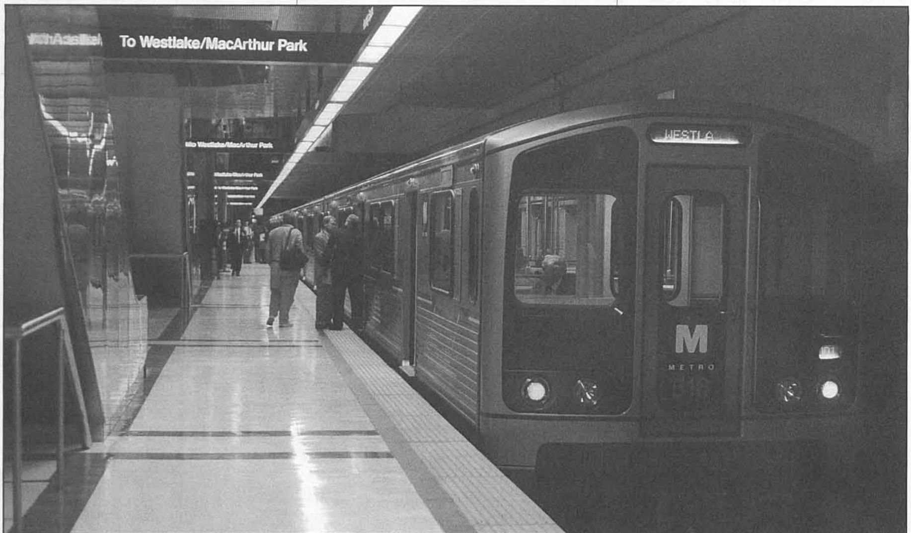
The Red Line's structural integrity passed two rigorous tests: a thorough examination by experts and an earthquake.
