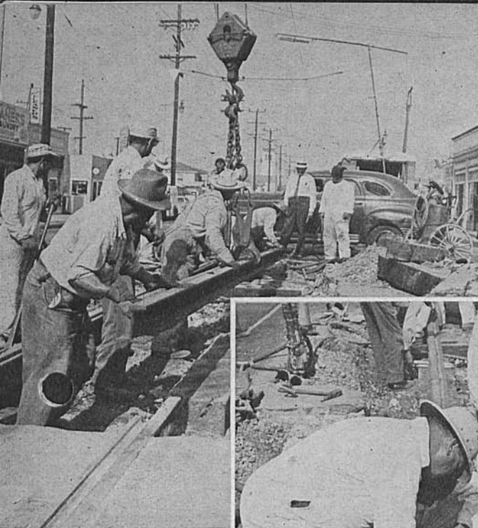
116-LB. RAIL, pre-cut to fit exactly, is swung into place . . .
