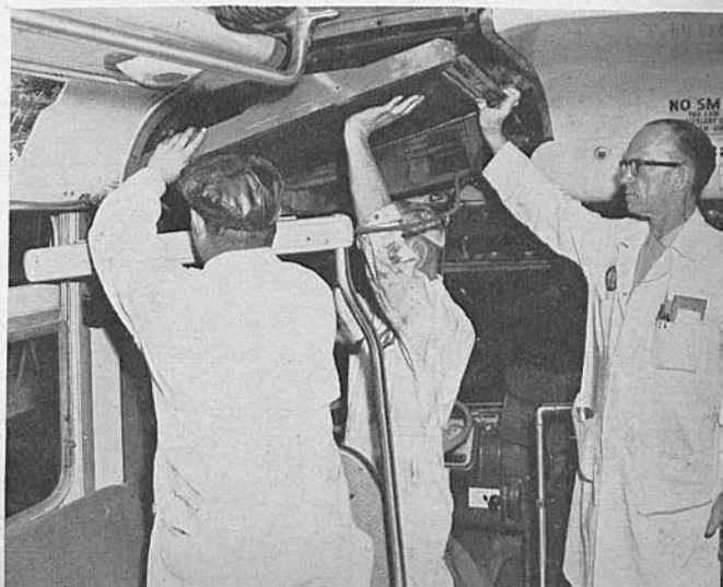
HUBERT DENNIS, second shift Foreman, right, supervises installation of new heater radiator in a 2800-class bus. Mechanics are Leonard J. Davis, left, and Herbert Fassbender. →
