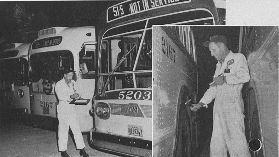
BEFORE DAWN at Redondo Terminal-Division each day, Mechanic Myron Lund checks defect cards (picture at left) on each of 14 buses to see if equipment needs mechanical attention before early morning pull-outs. He also inspects tires—fronts visually, rears by striking with hammer (picture at right)—to make sure there are no flats and pressure is up.
