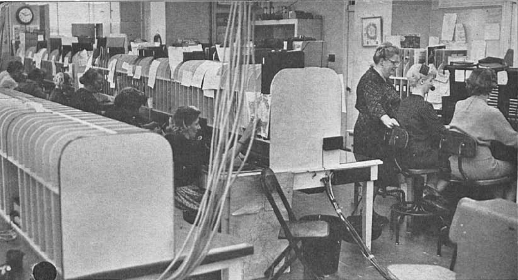
WORKING UNDER DIFFICULTIES —The crowded Information Department room shortly before the changeover to the new 28-position board partly shown in left foreground. Eight Information Clerks are shown working at the old 16-place board. At right, Assistant Supervising Telephone Operator Mae Ruffner, standing, observes girls working at the PBX switchboard.
