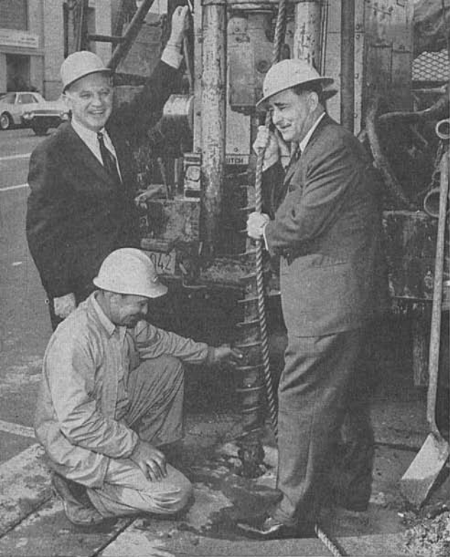
TWO WEEKS LATER (Jan. 23) drilling begins in the Beverly Hills area at Linden Dr. and Wilshire Blvd. Here Driller Bill Schwenk is "assisted" by N. R. Dumont, MTA Board member, left; and Jack Freeman, Mayor of Beverly Hills, right.
