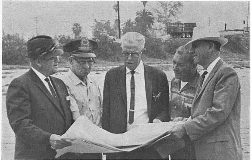
TENTATIVE PLANS for new garage are examined on the new site by, from left, Assistant General Manager M. Edwin Wright; Supervisor F. G. Cook, Mechanical Engineer D. E. Dent, Riverside Foreman J. W. Witt, and Superintendent of Property Maintenance L. C. Thompson.
