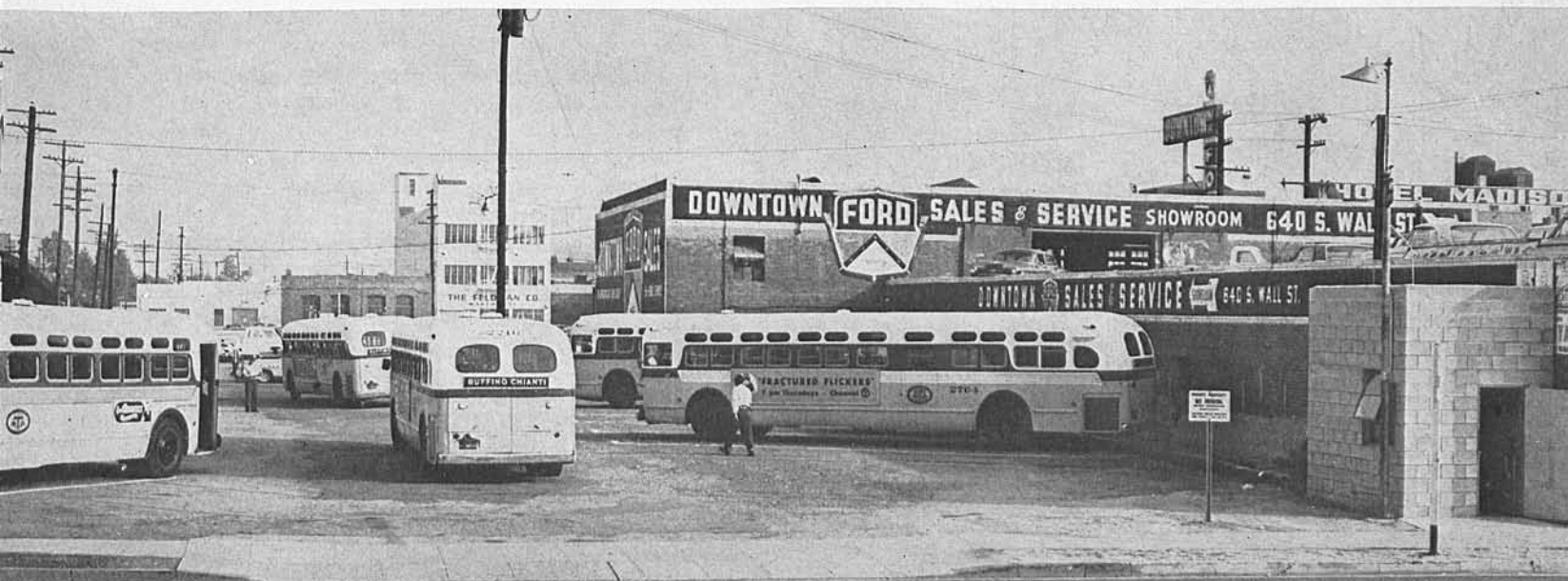
TERMINAL 17 , formerly known to most as the Maple Ave. Lot, is now used for storage of extra coaches which may be needed as doubles, etc., at the Main St. Station (Terminal 16). Note the new Service Director's building at right. In photo at right, Extra Service Director Tory Davidson, center, stands beside the new Service Director's building and checks coaches on the lot. Surrounding him are, from left, Operators G. J. Benchener, B. B. Brinker, J. H. Edwards, A. M. Botts, awaiting runs.
