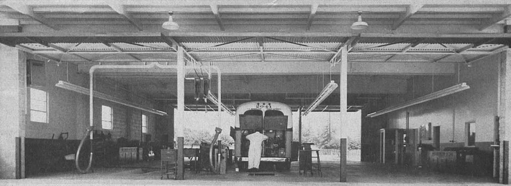
GARAGE INTERIOR , showing Mechanic Mike Duvigneaud working on a bus over one of the two pits. Note overhead doors (automatic) at each end; overhead oil and water reels; exhaust eliminators (curved pipe); fluorescent lighting.
