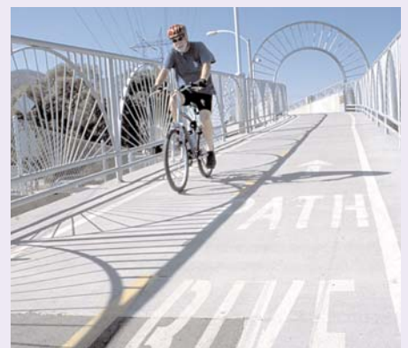
Spanning the Los Angeles River at Los Feliz Boulevard, the Alex Baum Bicycle Bridge is a link in the Los Angeles River Bike Path. One of hundreds of “Call for Projects” transportation projects in part funded by MTA, the bridge opened in May.
