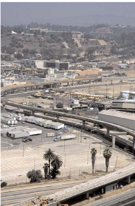
Trips to and from downtown Los Angeles will include 1/2-mile aerial guideway segment between Union Station and Chinatown.
