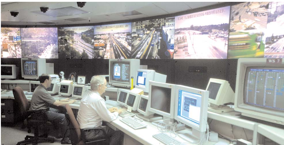
The Automated Traffic Surveillance and Control (ATSAC) center monitors traffic and controls signals.
