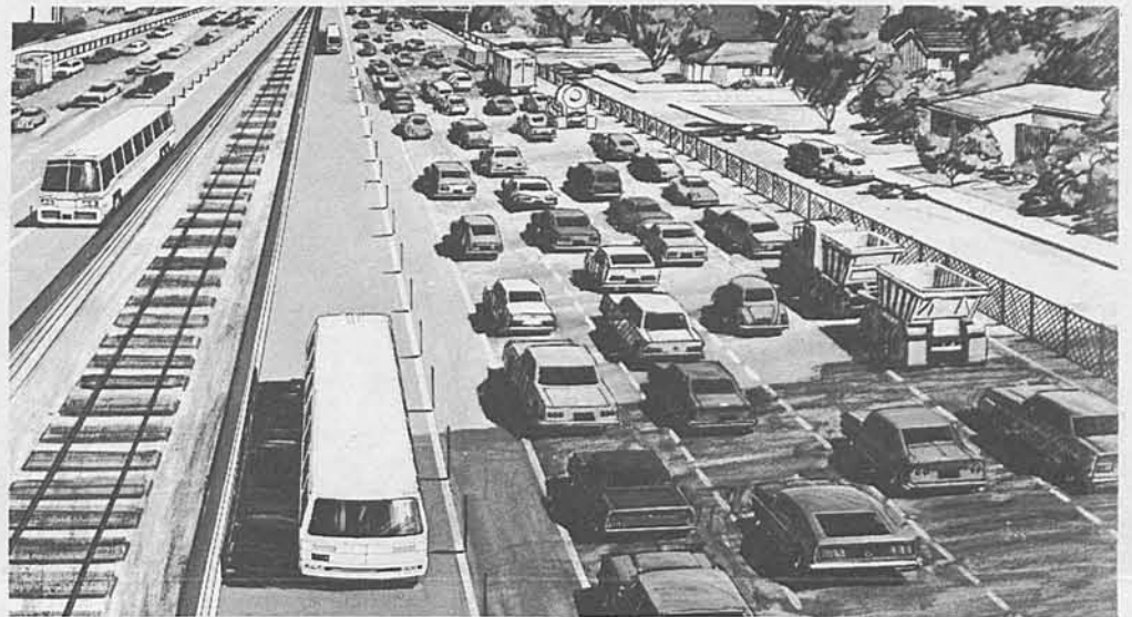
SIXTY-FIVE MPH THROUGH SIGALERT COUNTRY —Traffic-trapped motorists will find RTD Busway Flyers passing them up when District's exclusive express busway goes operational in fall, 1972. Comfortable air conditioned buses will travel 65 miles an hour between El Monte and Los Angeles on exclusive lanes in the center and alongside the San Bernardino Freeway. Travel time between the two cities has usually been about 40 to 45 minutes. Busway Flyers will reduce that time to 18 minutes.
