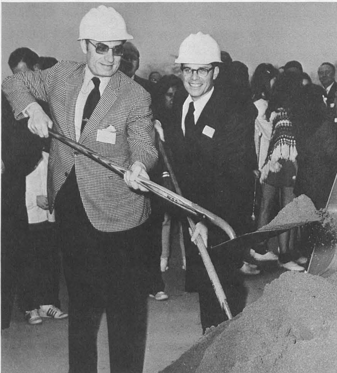
California Assemblyman Wadie P. Deddeh (D-Chula Vista) and RTD General Manager Jack R. Gilstrap "dig in" at groundbreaking ceremony commemorating the beginning of construction for RTD's exclusive express busway from El Monte to Los Angeles.
