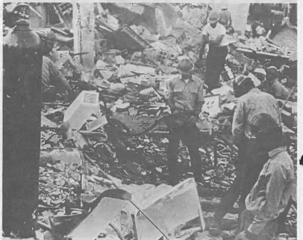
QUAKE AFTERMATH—Workmen pump air to victims under rubble of Veterans Hospital in Sylmar after the 1971 San Fernando Valley tremblor.
