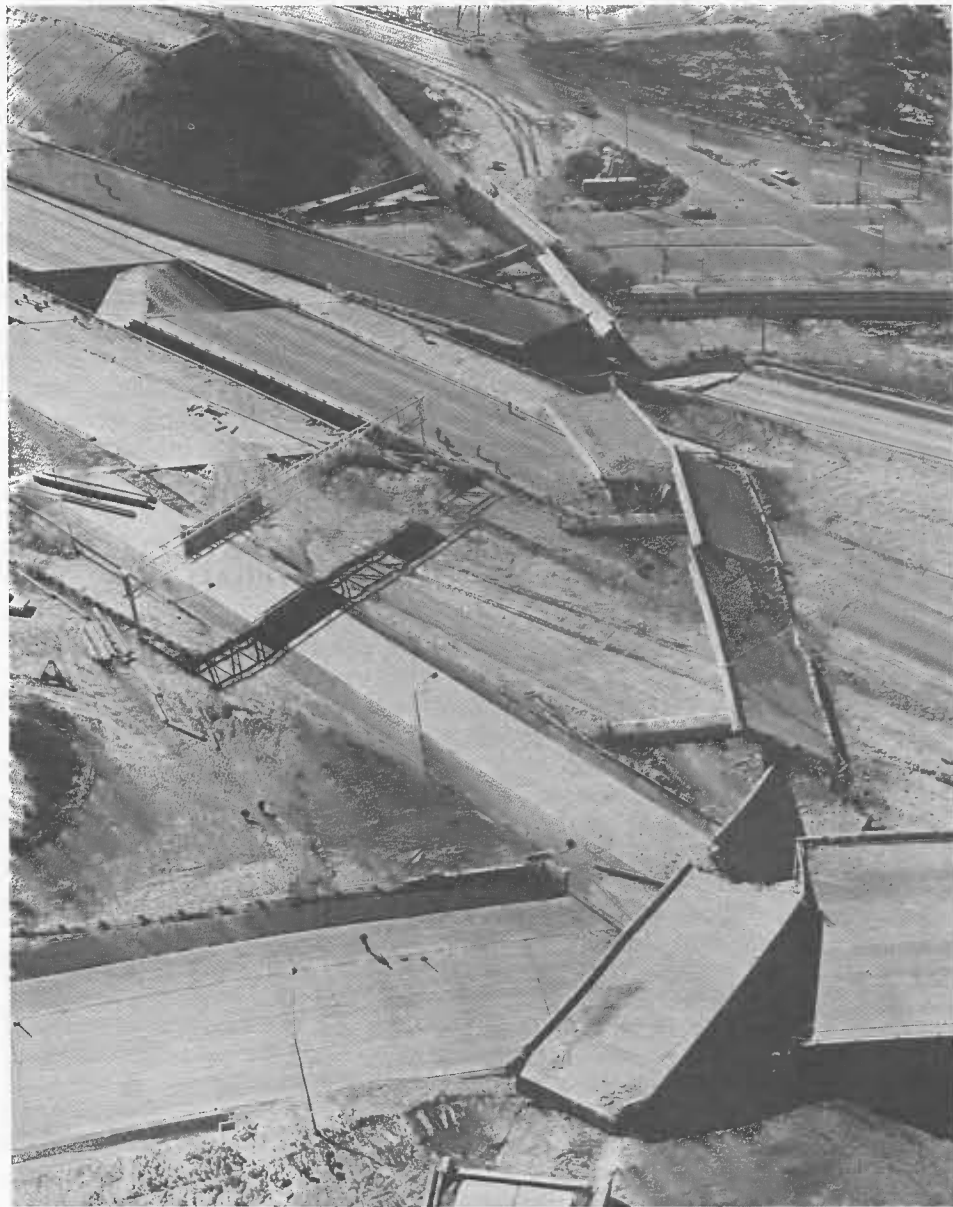
FREEWAY DEVASTATION —The 1971 San Fernando earthquake broke this overpass to the Golden State Freeway like a matchstick. Such destruction can bring transportation to a standstill and illustrates the necessity of preparing to be self-sufficient in the aftermath of a major quake. Quake damage can also cut off communications.
