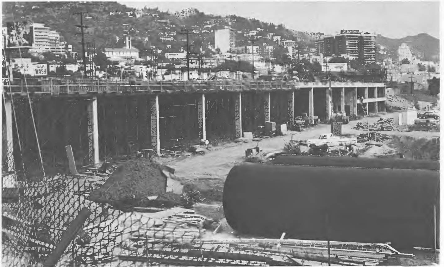
The combined transportation and maintenance building is 504 feet long and 80 feet wide. Shown above is only the ground level, on top of which will be two parking levels for both company and employee parking. The rear of the building faces Santa Monica Blvd.
