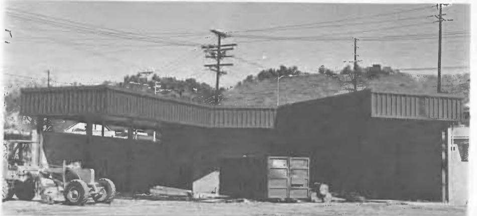
This is the front view of the tire maintenance and repair shop. The canopy will offer some protection from inclement weather for personnel changing tires. All the tires will be stored in this building.
