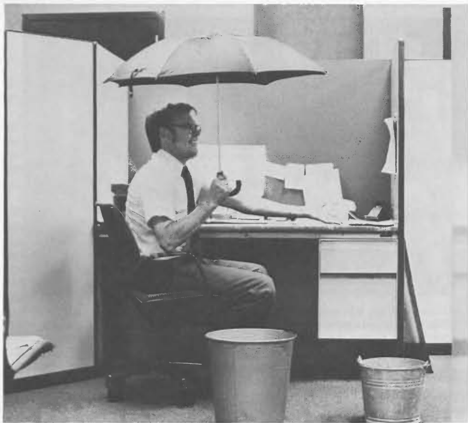
"RAINDROPS KEEP FALLING ON MY HEAD" wasn't really being hummed by Jack Penwell in Operations, but it would have been an appropriate tune. As the record rainfall continued to pelt the Southland, a few leaks were detected in the roof above his office inside the leased District headquarters building. However, with wastebaskets doubling as rain buckets, Jack weathered the storm in his usual goodnatured style.
