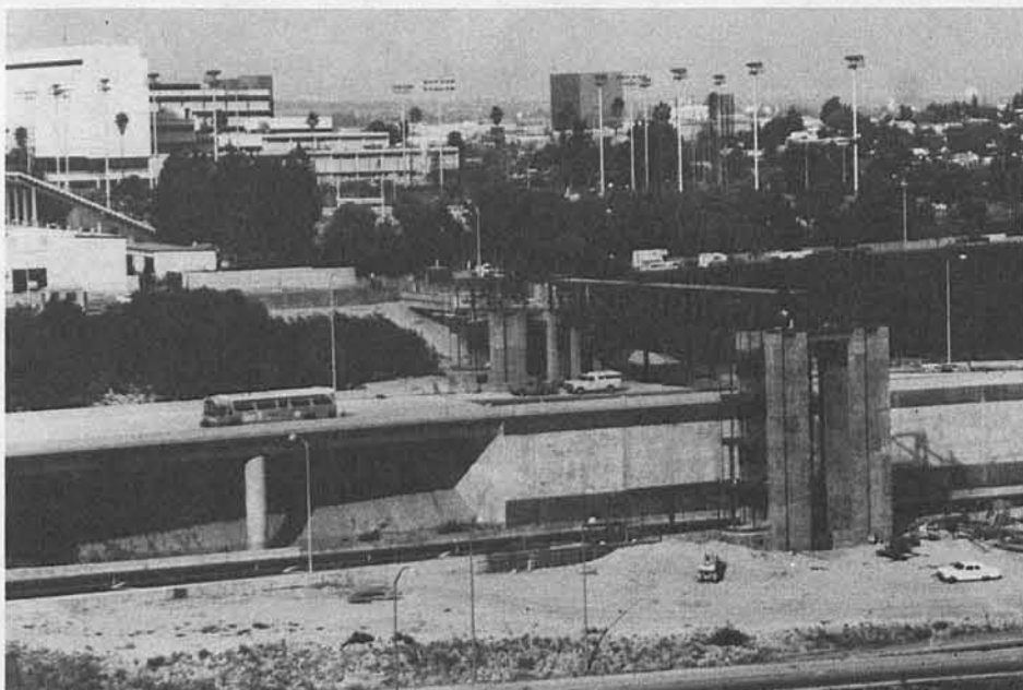
PROVING A POINT — Buses streak past peak hour traffic tie-ups in the special Busway lane (top photo). Service began five years ago this month with the University Station (above) still under construction.
